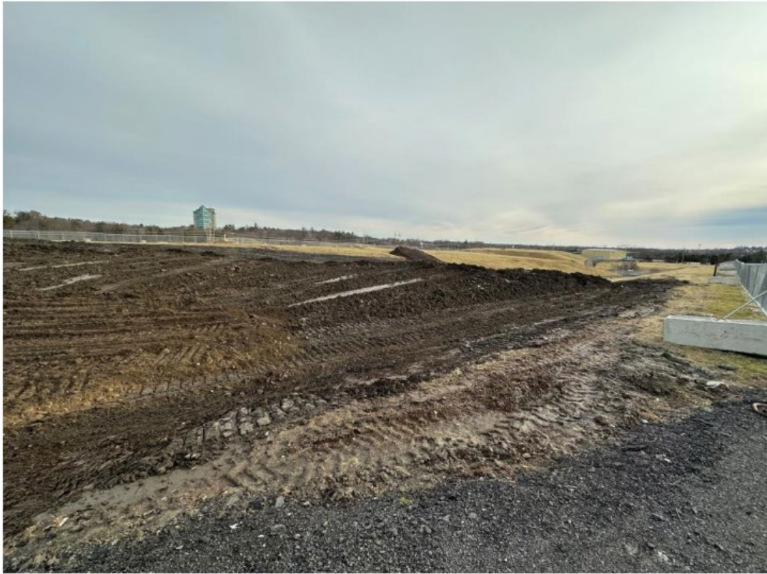
Figure 10. This is a photo of the Danvers Landfill project (photo shows progress on soil filling in Phase 1 area to support future solar development).
