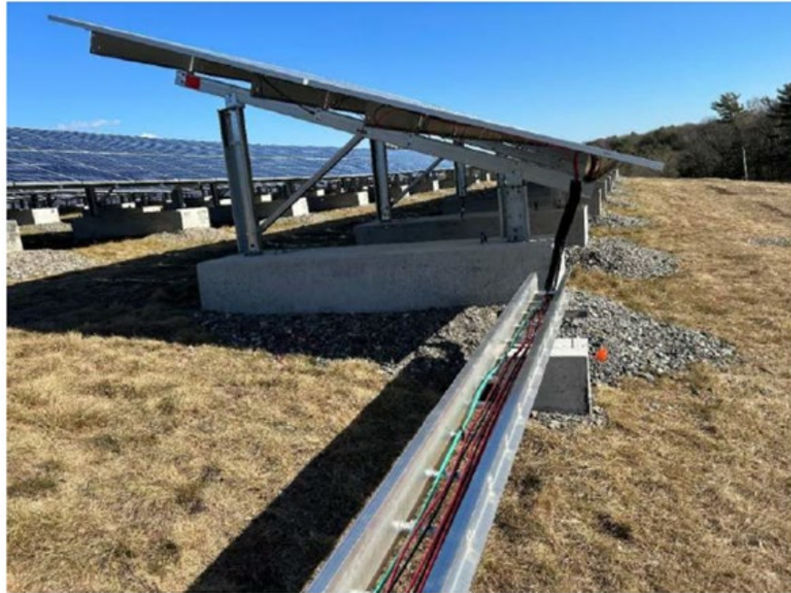
Figure 13. Cable tray installation at the Kingston Landfill. aboveground conduits are a typical design as MassDEP. It does not allow penetrations of a landfill final cover system.
