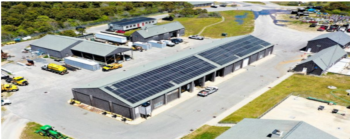
Surfside Wastewater Treatment Plant 104.4 kW Solar Array (Funded by Gap Energy Grant)
