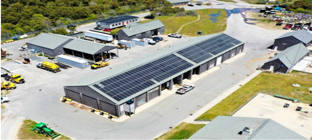
Figure 4. Surfside Wastewater Treatment Plant 104.4 kW Solar Array (Funded with Gap Energy Grant)
