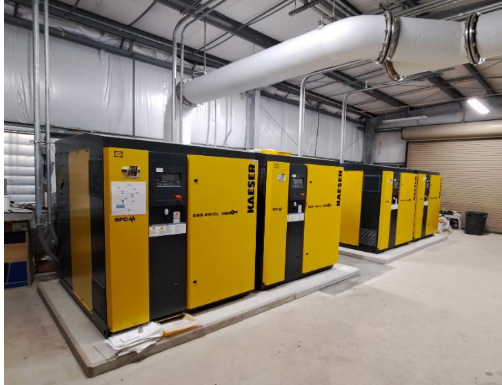
Figure 5: New Aeration Blower Equipment at the Ipswich Wastewater Treatment Plant
