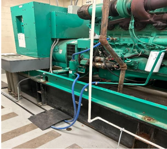
Figure 3: Emergency generator (left) and block heater for the emergency generator (right) at the West Gloucester Water Plant
