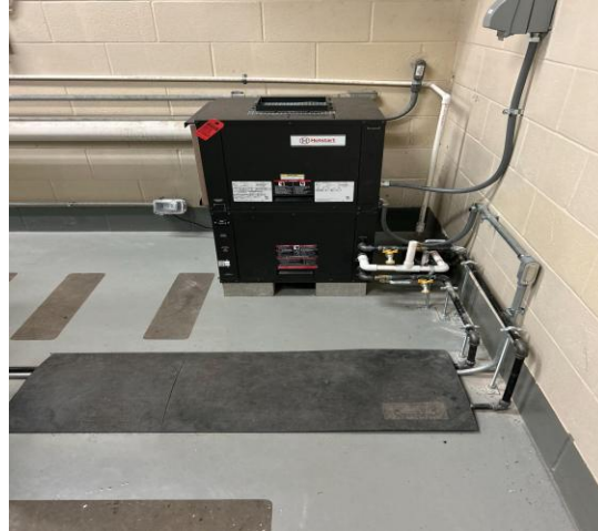
Figure 3: Emergency generator (left) and block heater for the emergency generator (right) at the West Gloucester Water Plant
