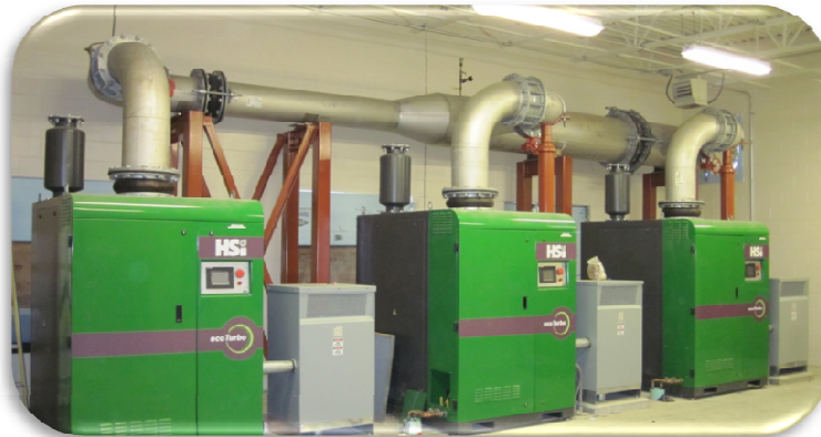
Aeration Upgrade - Diffused Air w / Turbo Blowers
