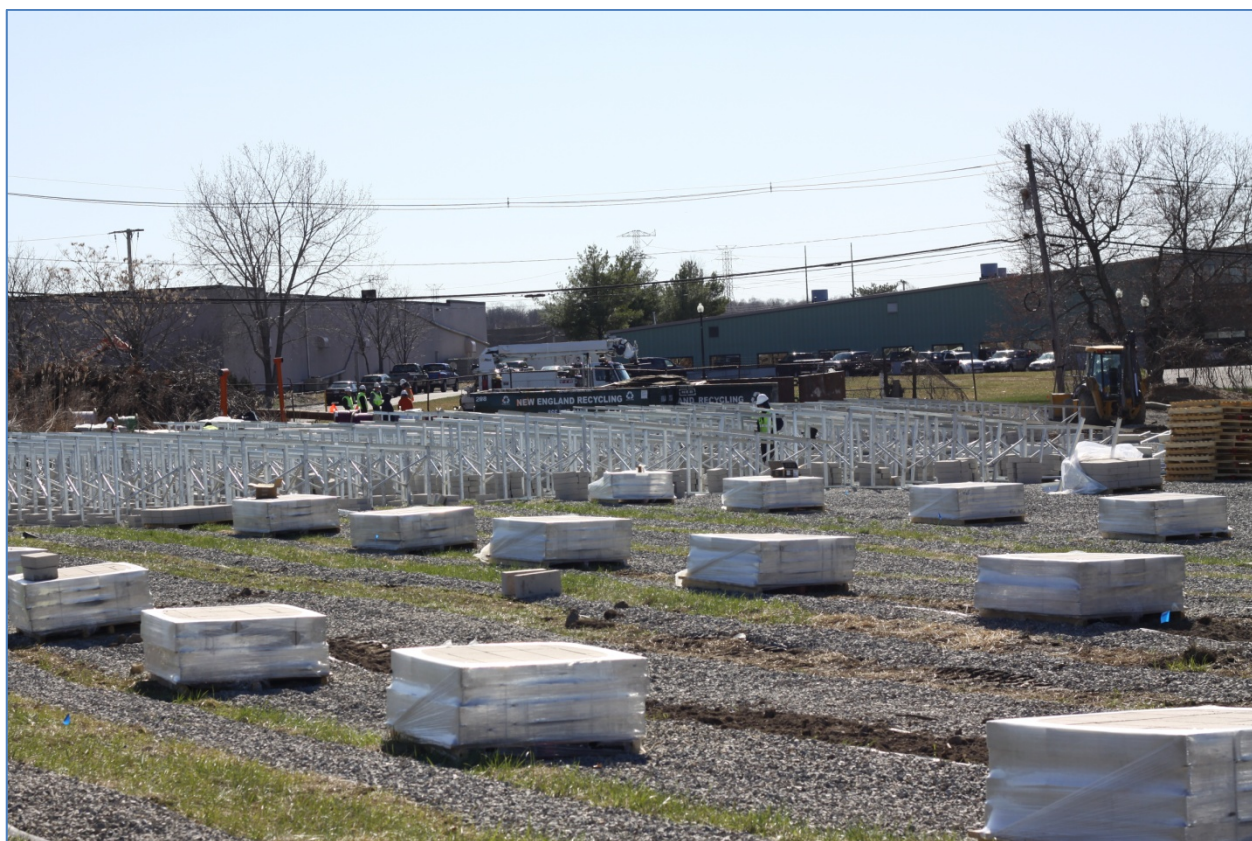
Solar Construction at Canton Landfill (6.7mw)
