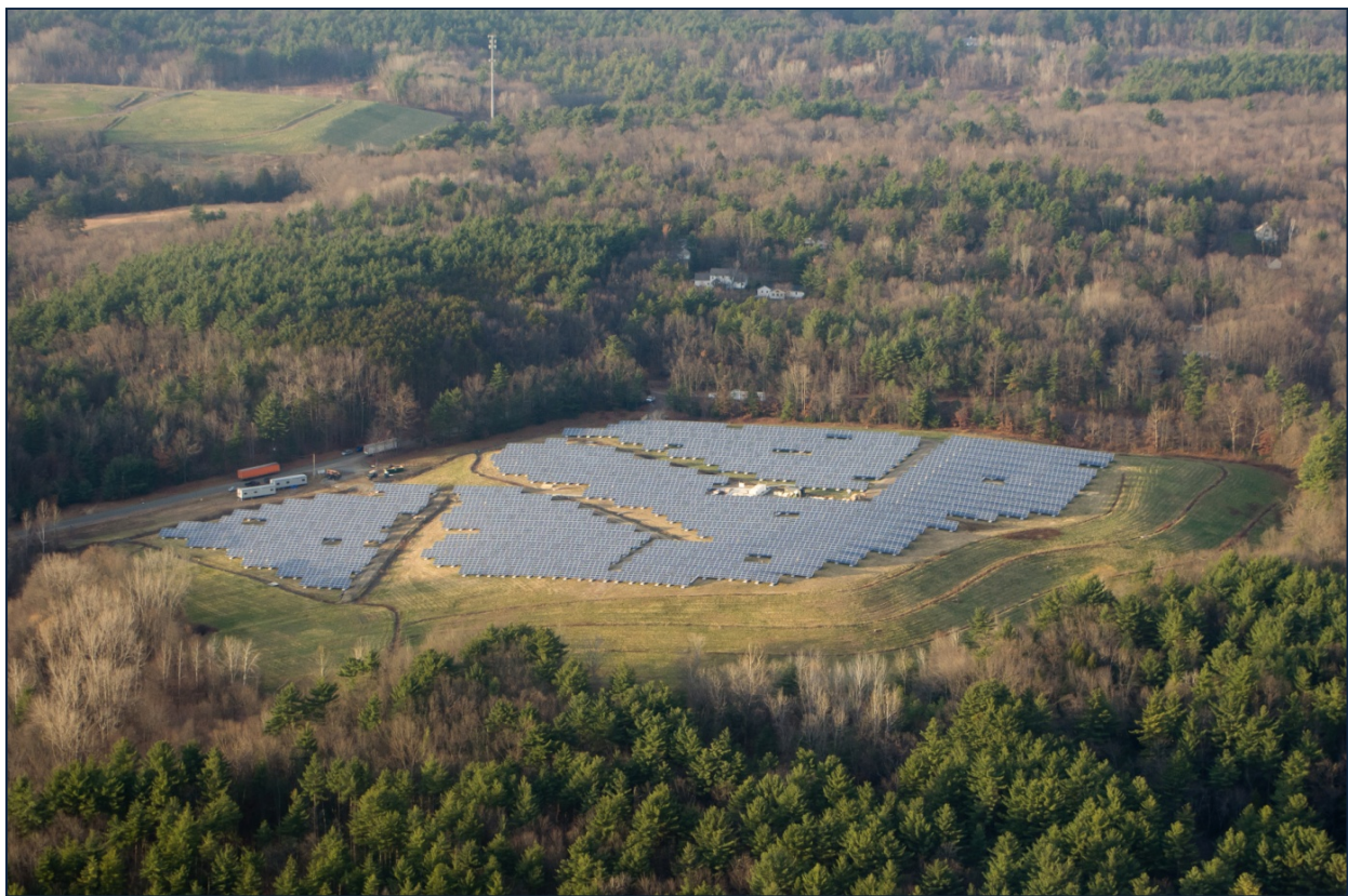
Easthampton Landfill Solar Project: 2.3 megawatts
