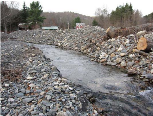
Left: Emergency work completed in the months following Tropical Storm Irene included extensive windrowing, as gravel and cobbles were excavated from the channel and piled as berms along Clesson Brook. Photo by Andrea Donlon. Right: Headcuts, or knickpoints, migrating upstream during high flow events represents vertical instabilities in the streambed initiated in the aftermath of Tropical Storm Irene. Photo by Nic Miller.
