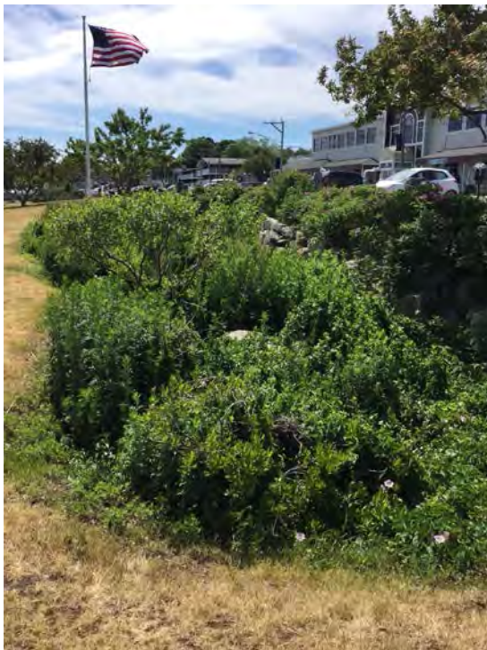
Green grass indicates overflow from bio. Erosion on other side of sidewalk where overland flow discharges to sea wall.
