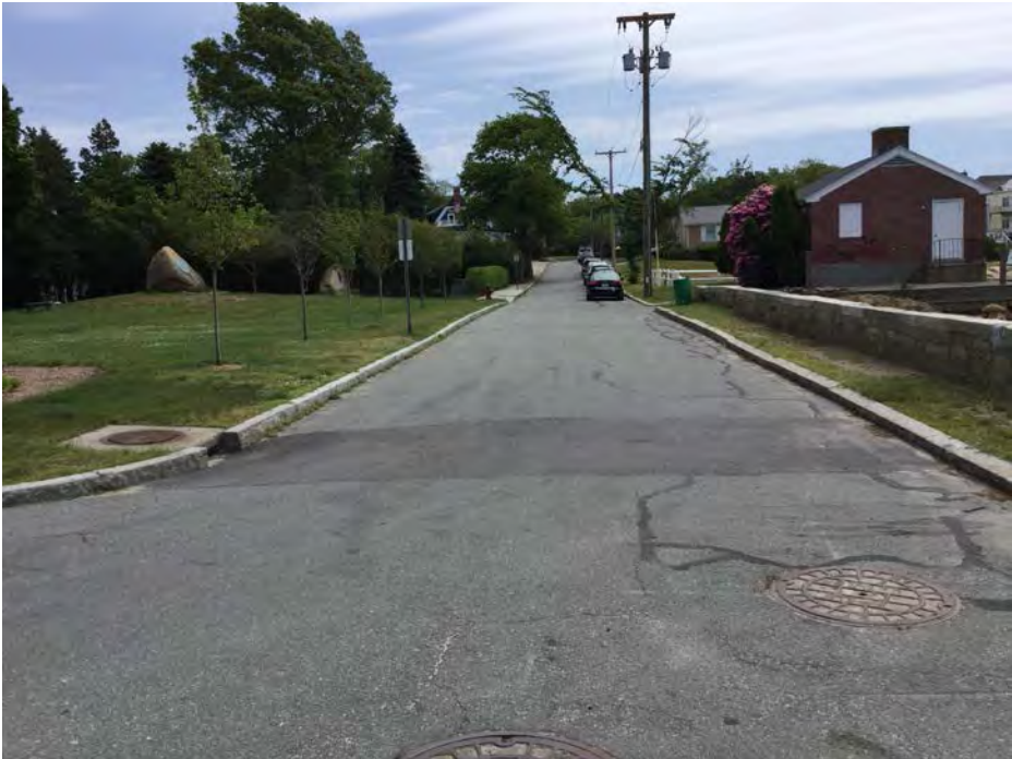
Drains to catchbasin at rain garden outlet.
