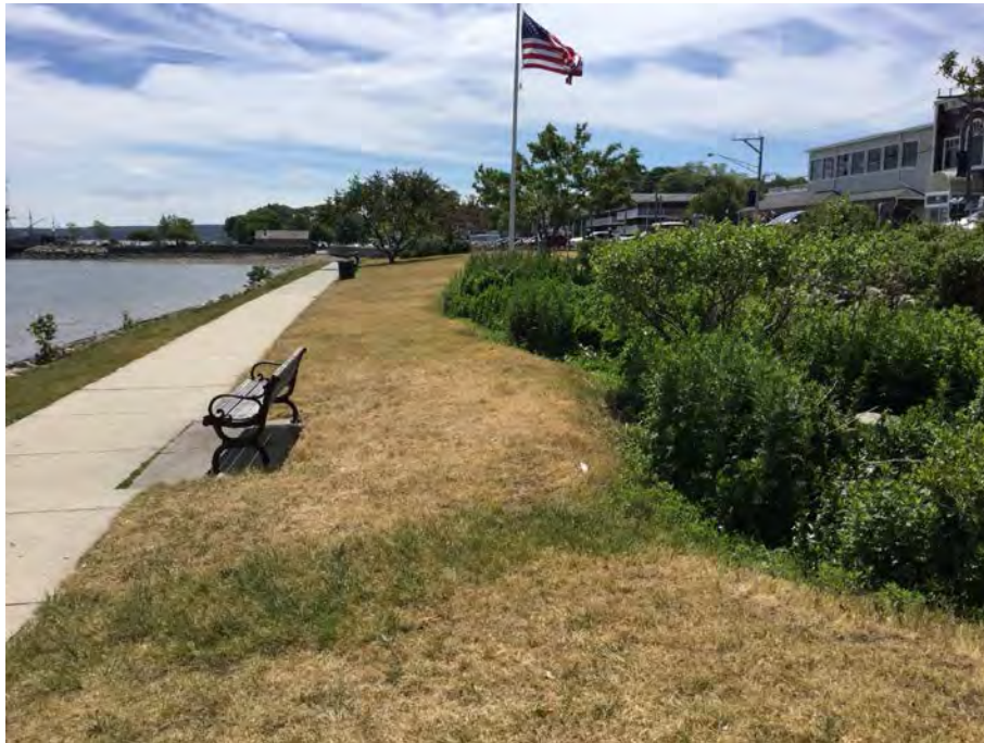
Green grass indicates overflow from bio. Erosion on other side of sidewalk where overland flow discharges to sea wall.
