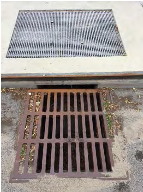
Site 11B, Dover Street. Trees not installed.
