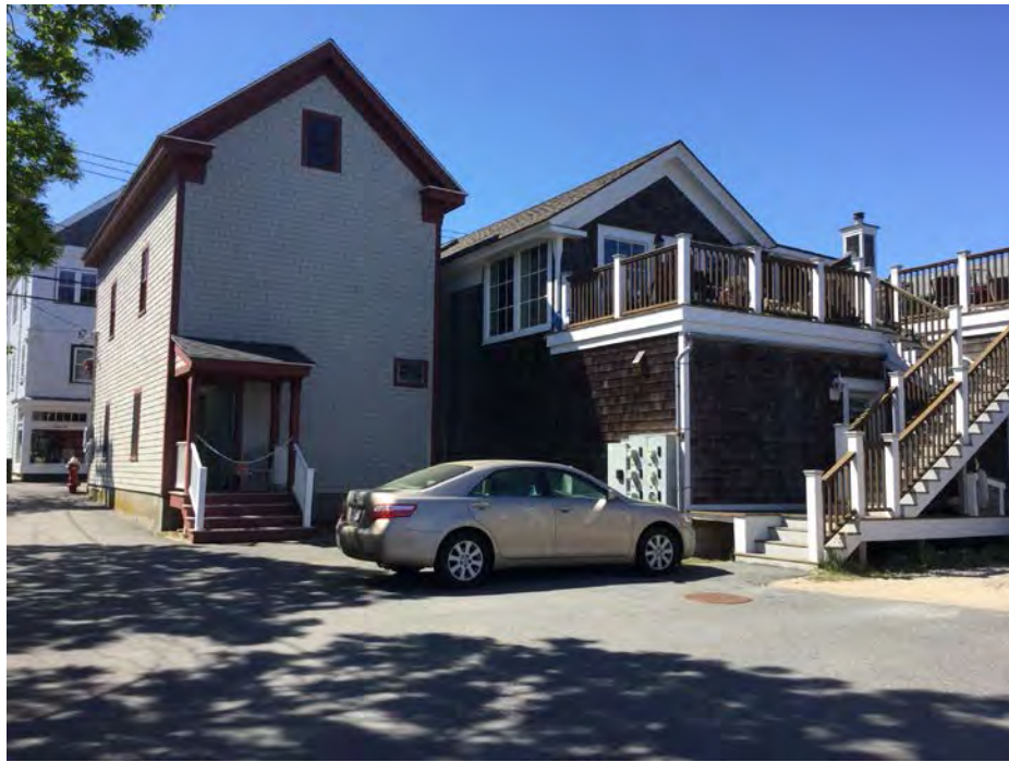
Two buildings in drainage area to practice.
