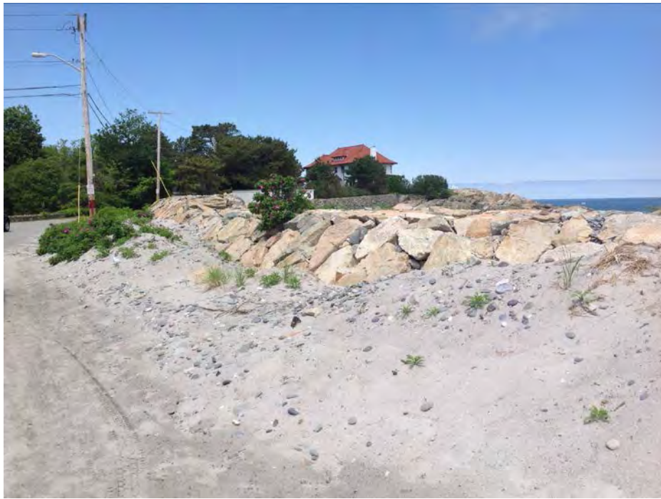
Sand appears to wash over lower section of sea wall, across Atlantic Ave. from BMP.
