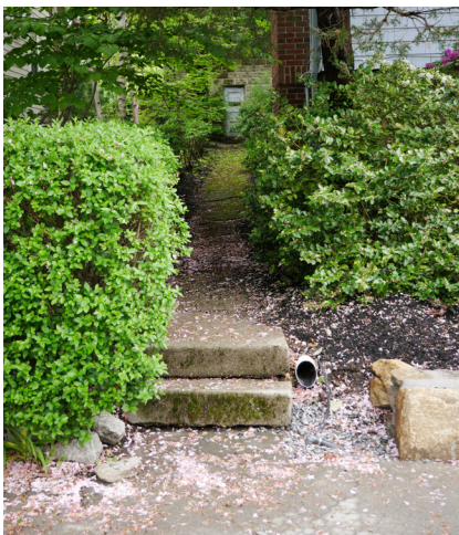
Roof runoff directed into permeable area.
