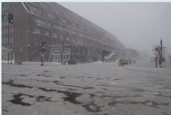
Flooding in Boston during Storm Grayson (January 4, 2018).
