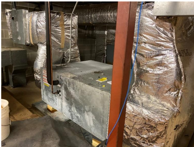
Photo 2 – Air Handler AHU-2
