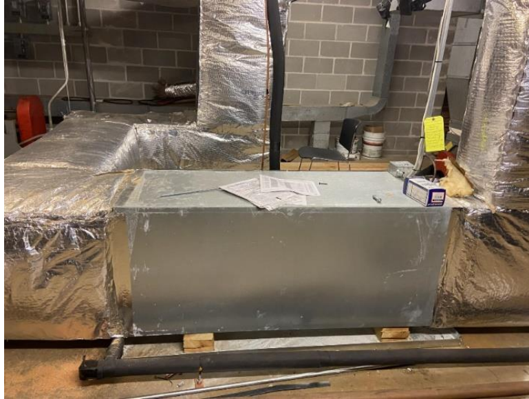
Photo 1 – Air Handler AHU-1
