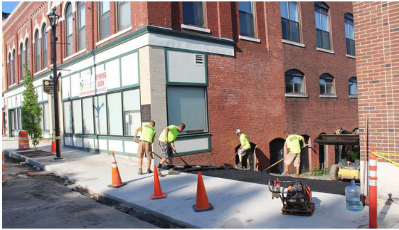
Installation of New Sidewalks and street furniture in Clinton
