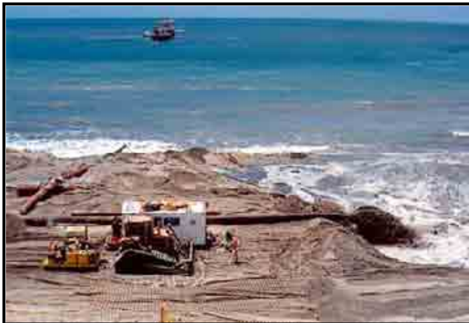
Figure 6-1. Beach nourishment project under construction.
