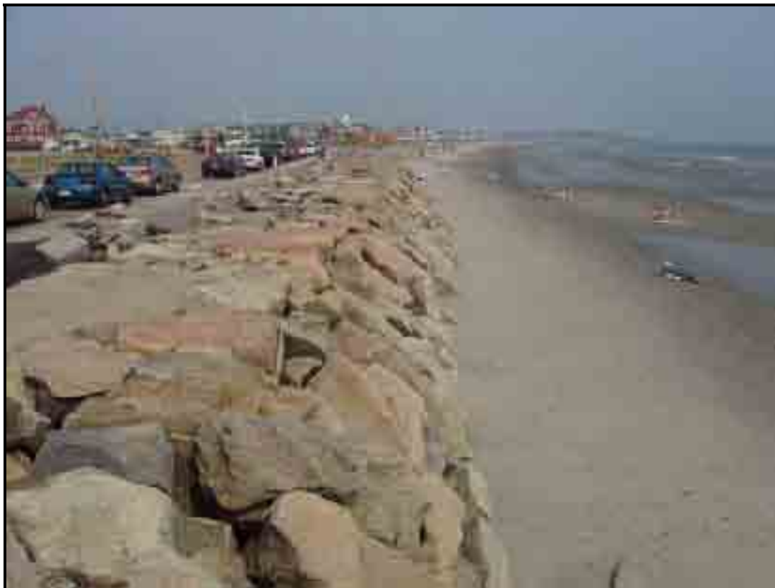
Figure 6-7. Revetment located along the DCR portion of Nantasket Beach.
