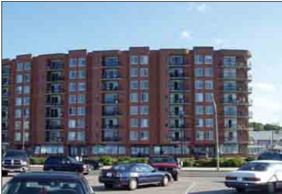
Figure 7-25. Ocean Place Condominiums.
