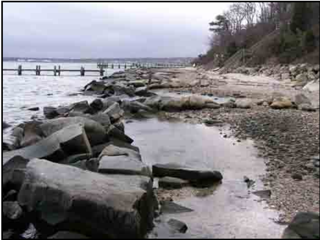
Figure 6-4. Example of a perched beach in Martha's Vineyard, MA. The perched beach has eroded behind the sill and is in need of replenishment.
