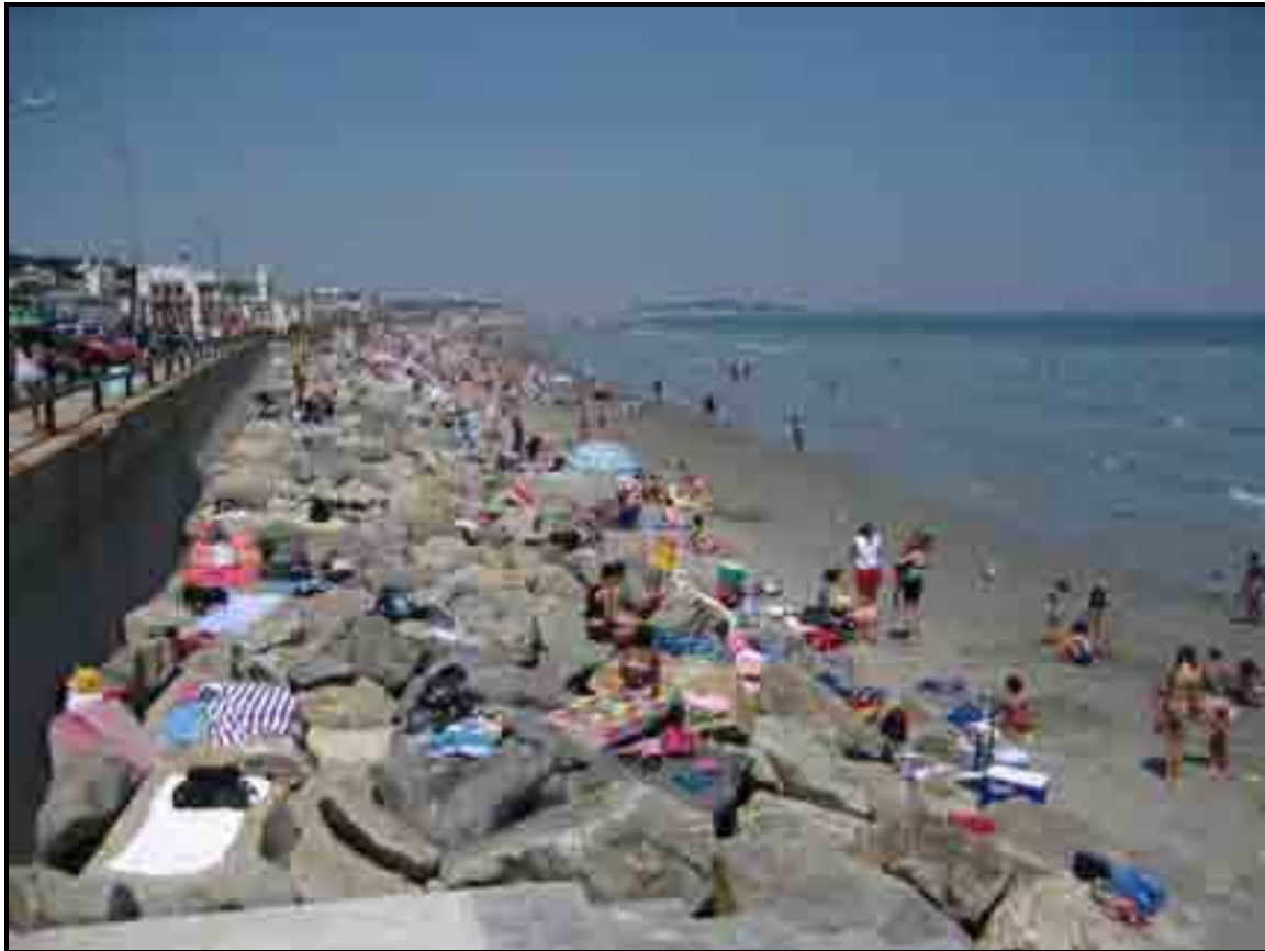
Figure 6-10. Seawall toe protection along the southern section of the Nantasket Beach Seawall.
