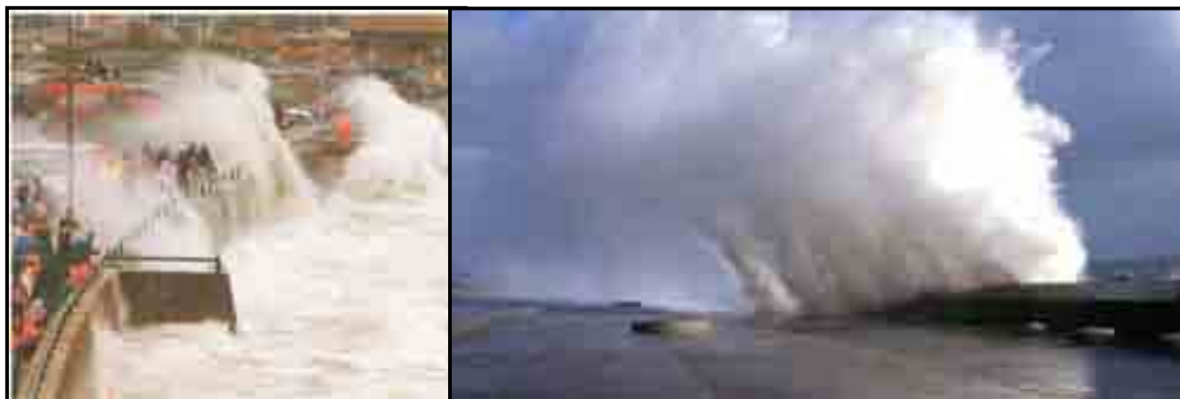
Figure 7-4. Examples of wave overtopping at seawall structures.
