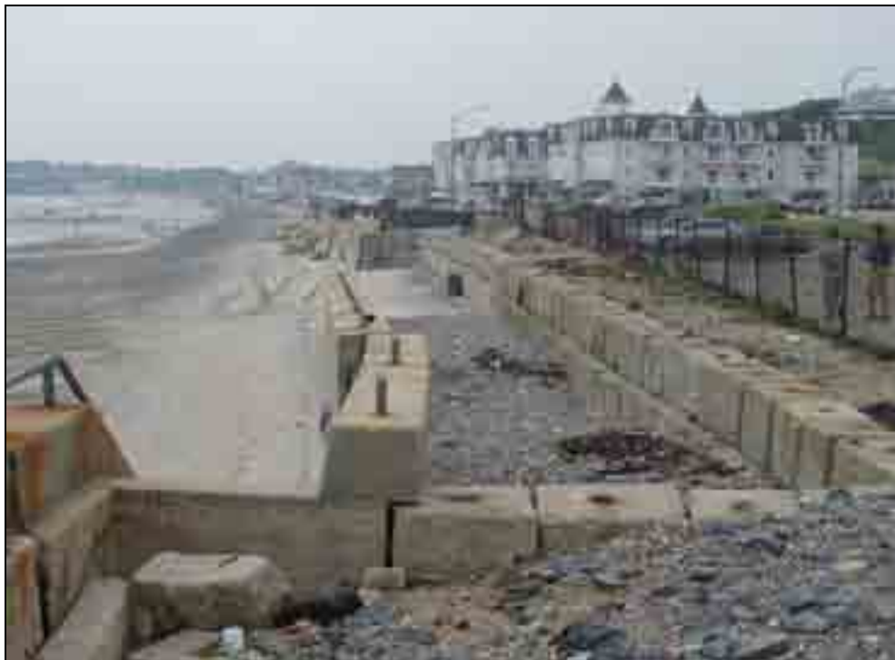
Figure 7-23. Damaged beach section along the northern section of the seawall. The seawall failed in 1991; it was repaired by 2006.
