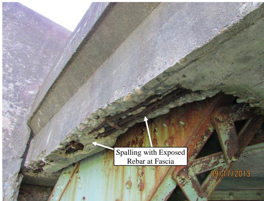
Figure 8.7 Spalling with Exposed Rebar at Fascia
