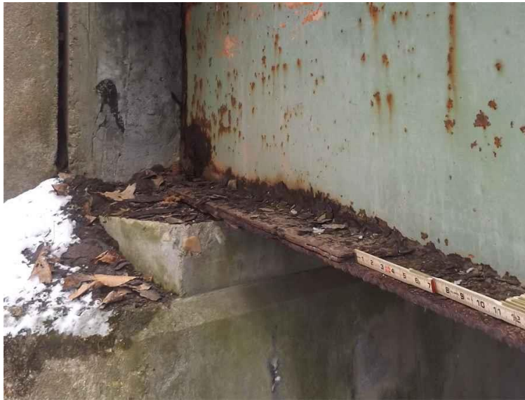
Figure 4.5 Typical Paint Failure and Steel Deterioration
