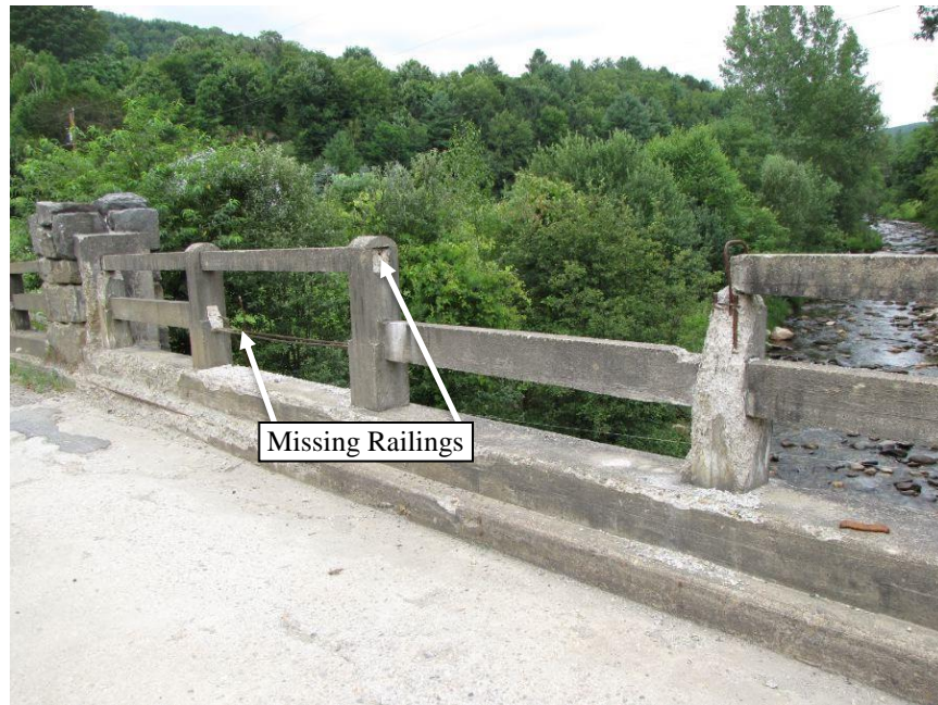
Figure 5.5 Missing Railings with Exposed Rebar
