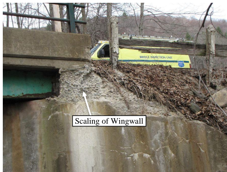
Figure 2.8 Scaling at the Southeast Wingwall
