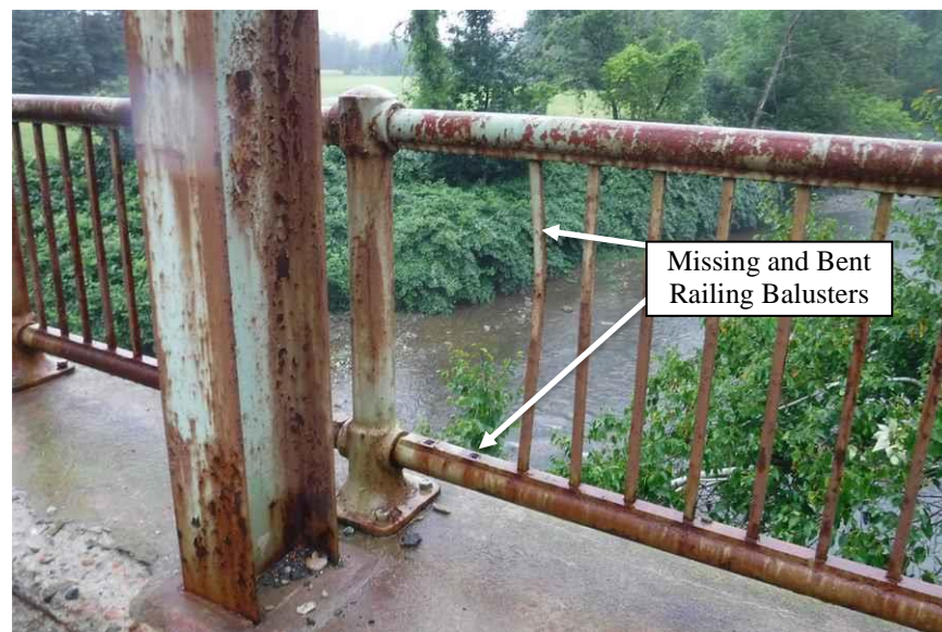
Figure 8.8 Missing and Bent Railing Balusters
