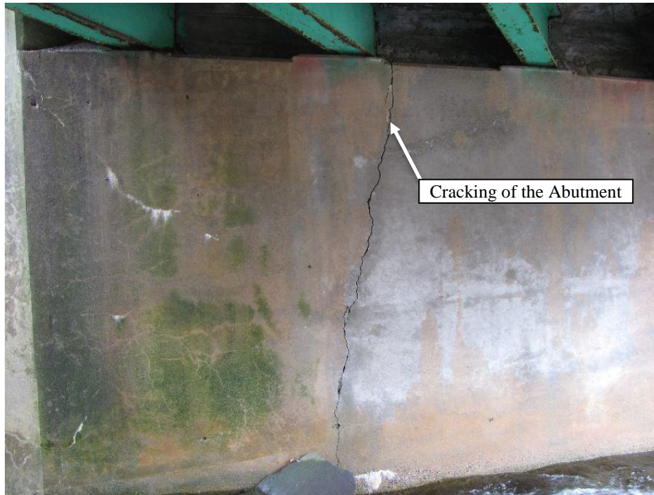
Figure 2.9 Cracking at Abutment
