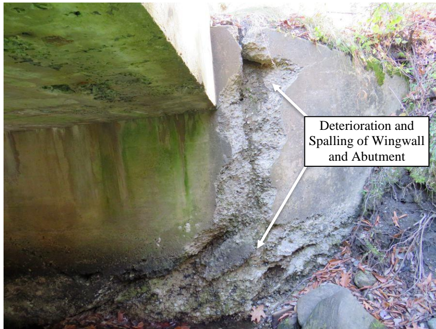
Figure 7.3 Deterioration and Spalling at the Southeast Wingwall and Abutment
