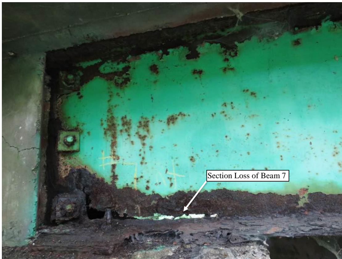
Figure 2.3 Beam 7 Section Loss
