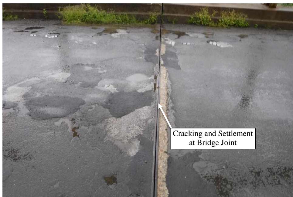
Figure 8.3 Cracking and Settlement at Bridge Joint
