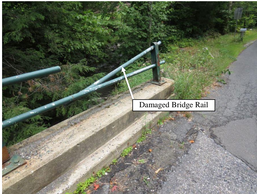
Figure 6.5 Damaged Bridge Rail
