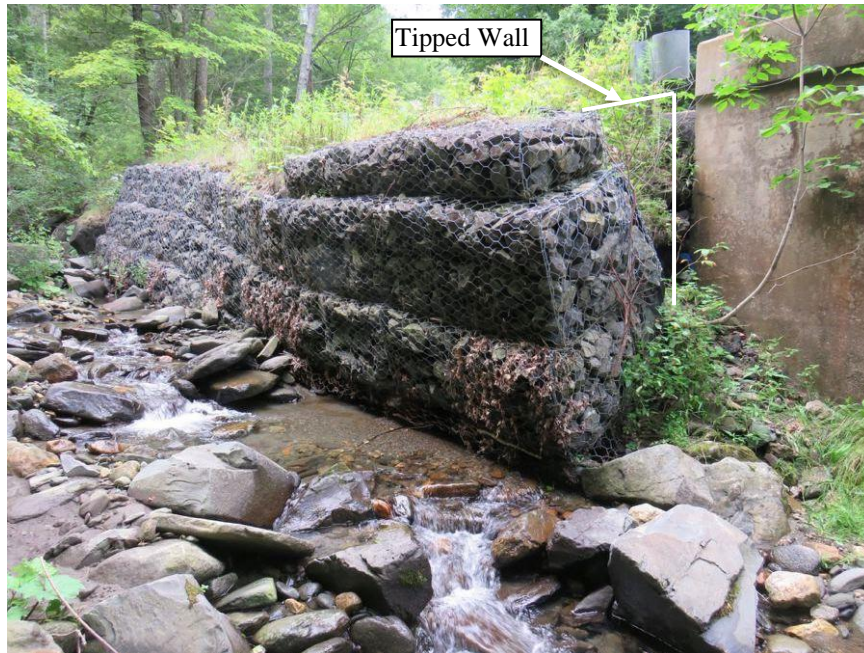
Figure 6.3 Southwest Gabion Wall Tipping and Falling
