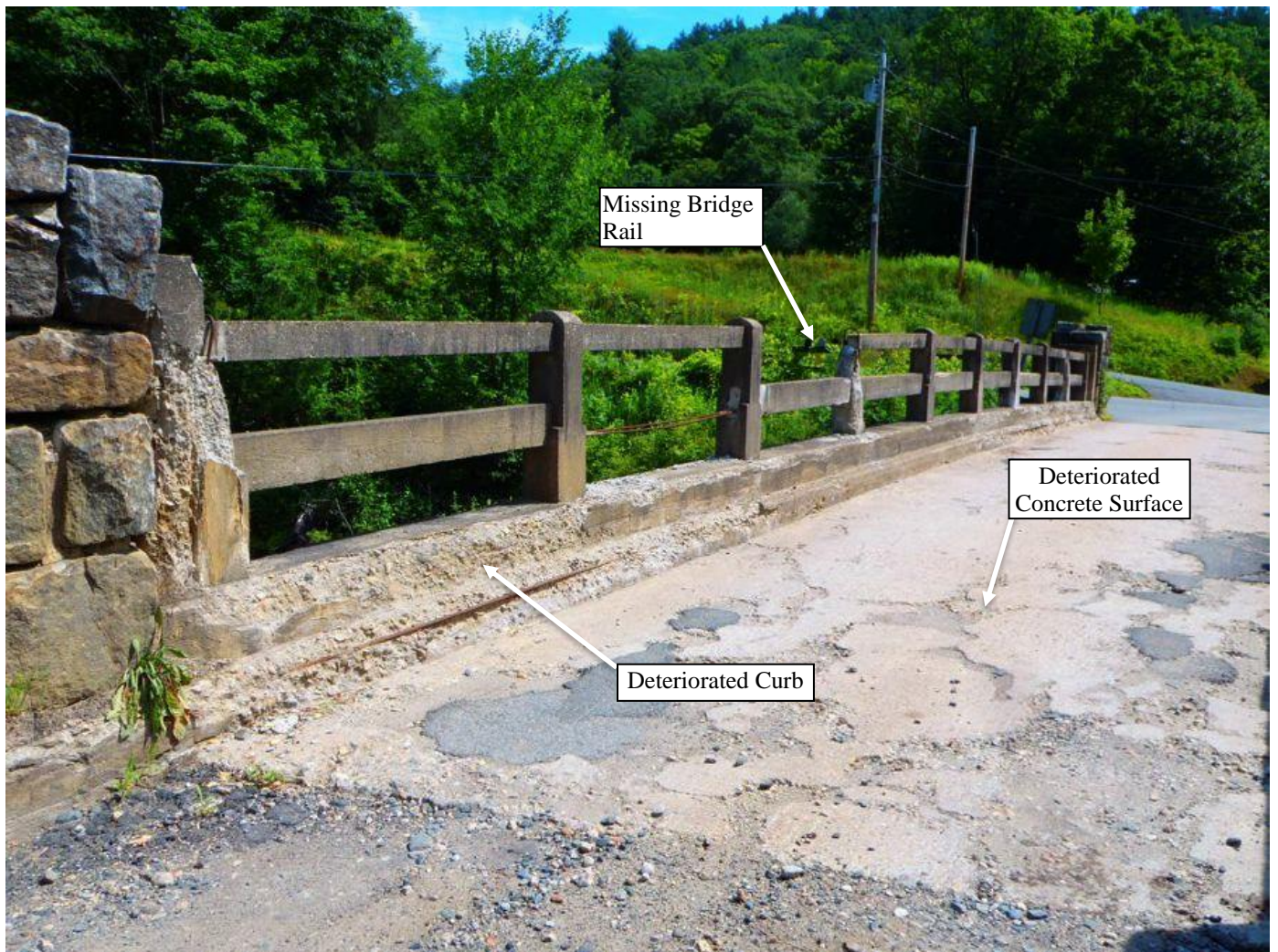
Figure 5.4 Deteriorated Railings and Curbs
