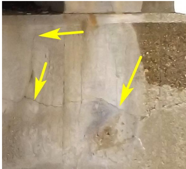
Figure 4.6 Cracking at the East Abutment
