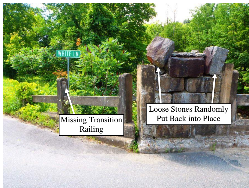
Figure 5.6 Railing Transition with Loose Stones
