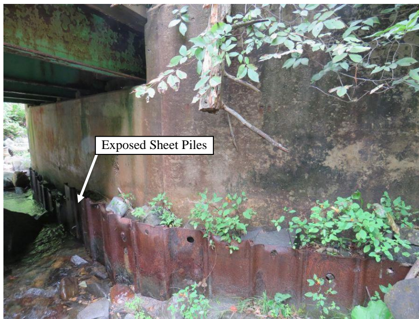
Figure 6.4 Sheet Piles at the East Abutment
