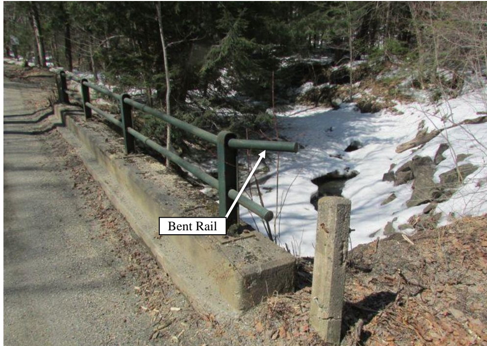
Figure 10.3 Bent Rail at Northeast Approach
