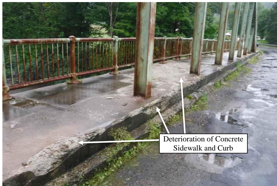
Figure 8.5 Deterioration to Concrete at Sidewalk and Curb
