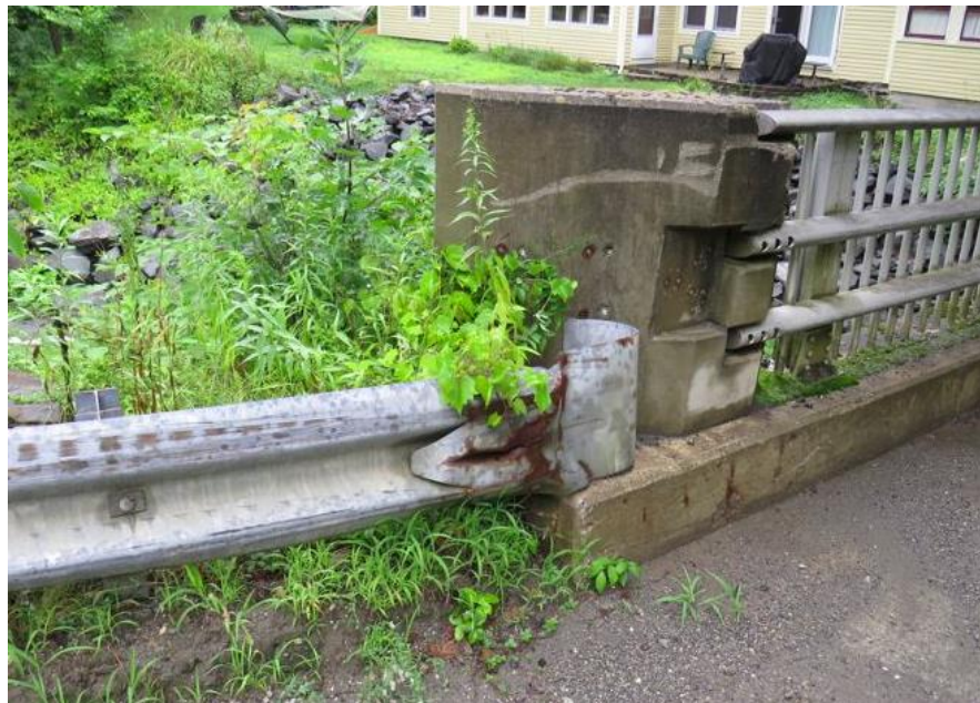
Figure 3.6 Typical Guardrail at Transition
