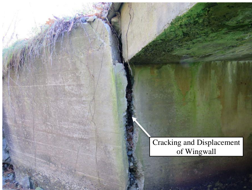
Figure 7.4 Cracking and Displacement at the Northeast Wingwall
