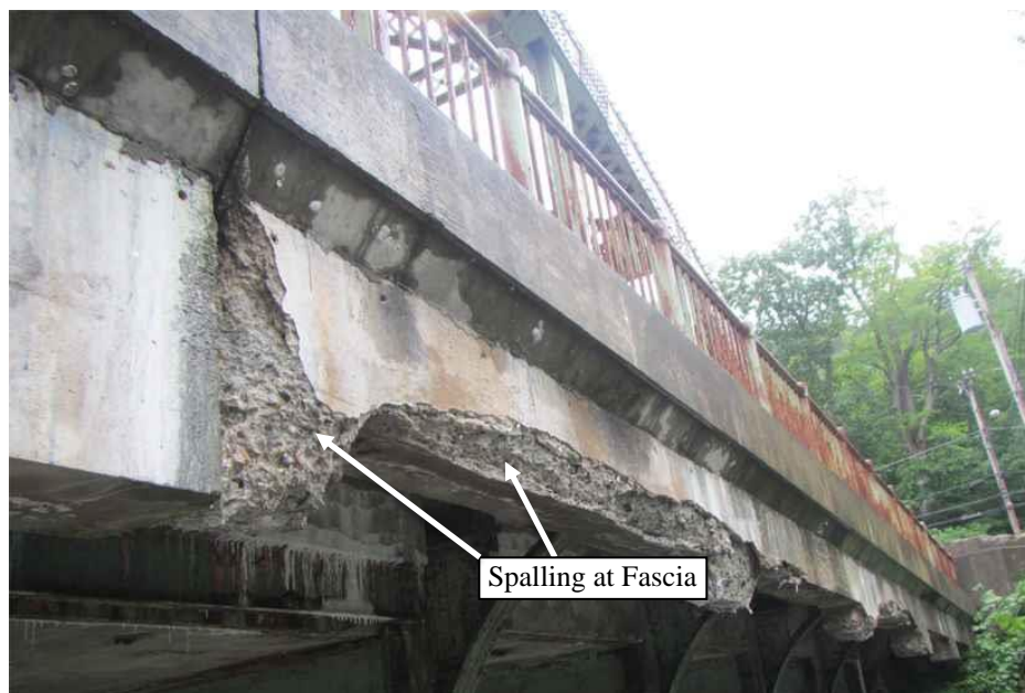
Figure 8.6 Typical Spalling at Fascia
