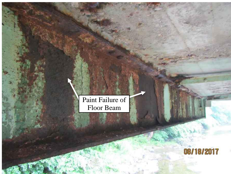
Figure 8.10 Typical Paint Failure to Floor Beam
