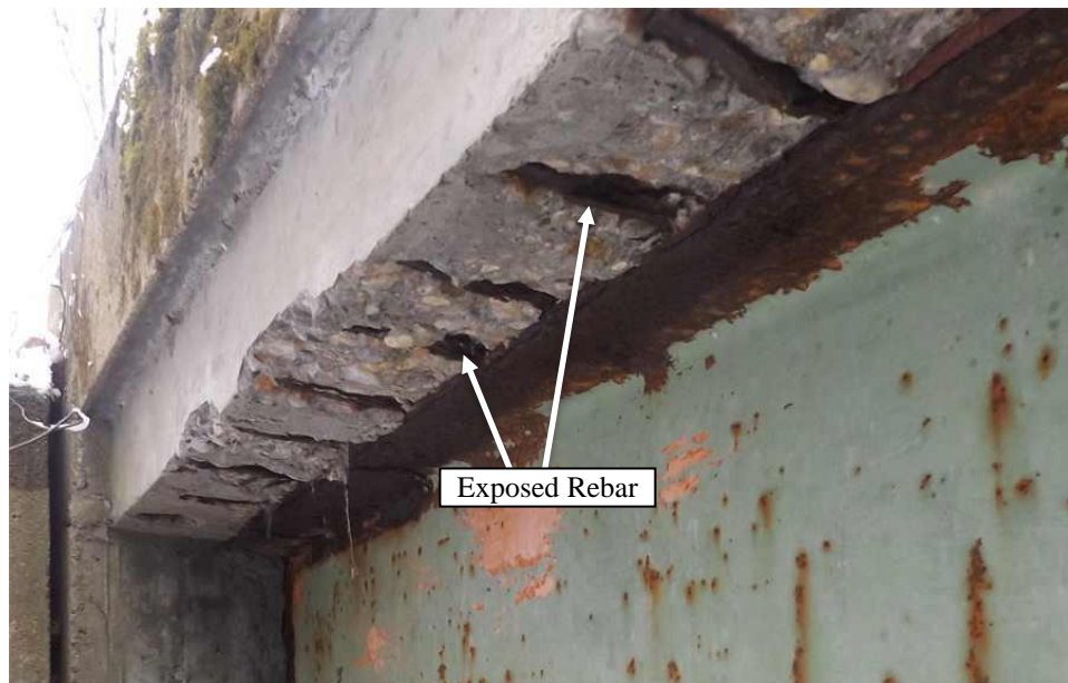
Figure 4.3 Spalling and Exposed Rebar at Overhang
