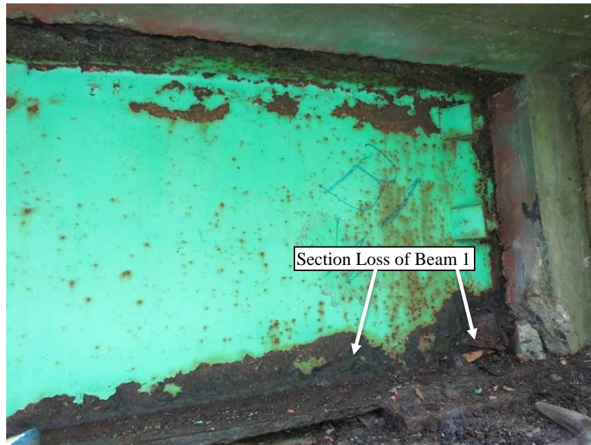
Figure 2.5 Beam 1 Section Loss
