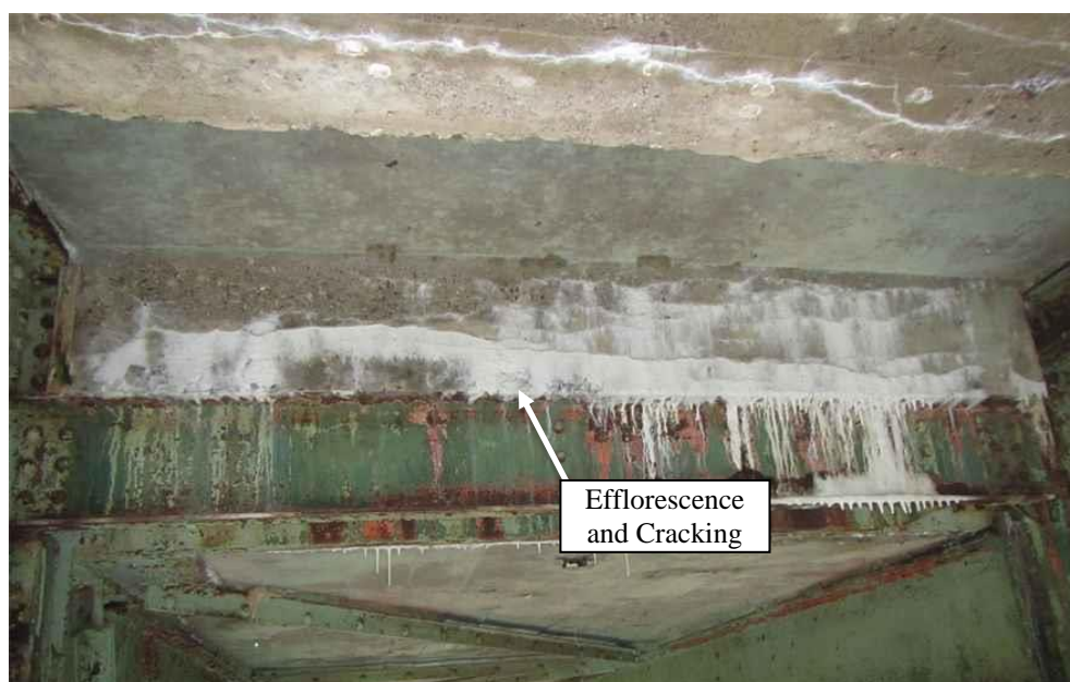
Figure 8.4 Efflorescence and Cracking Under Sidewalk
