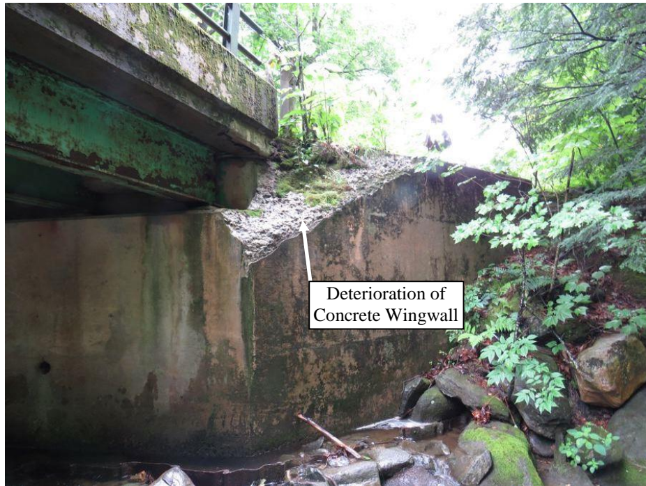
Figure 10.4 Typical Concrete Deterioration to South Wingwall
