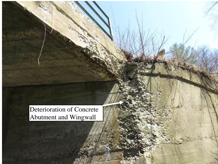
Figure 1.6 Typical Concrete Deterioration
