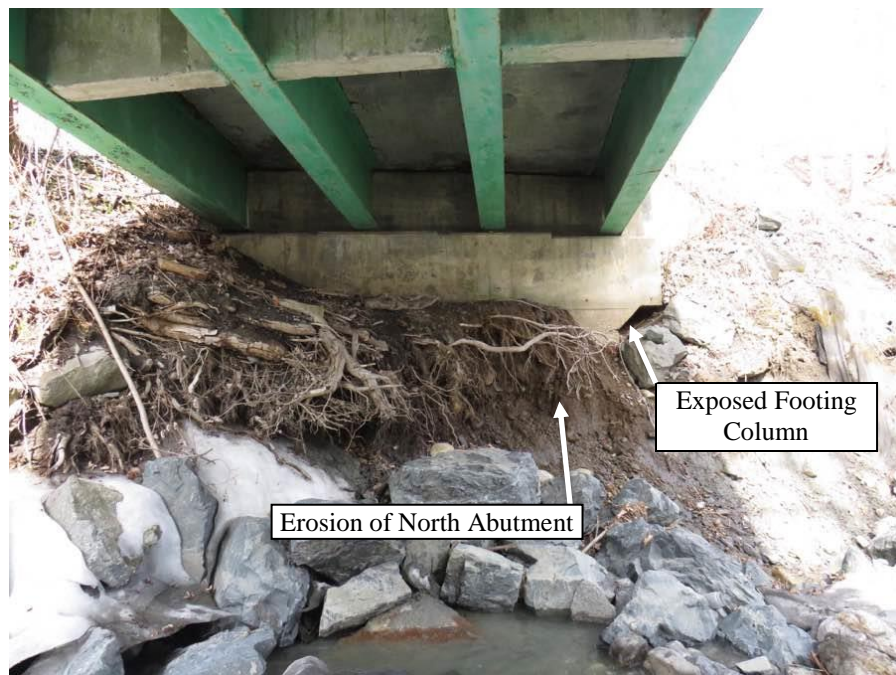
Figure 3.4 Erosion and Exposed Footing Column at The North Abutment
