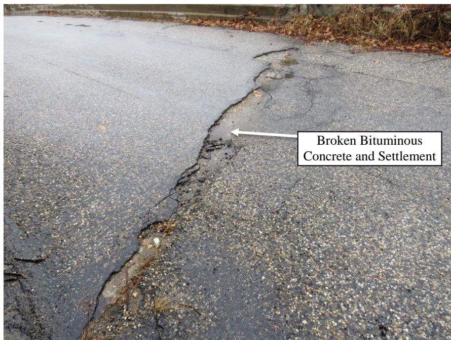
Figure 9.4 Broken Bituminous Concrete and Settlement at Bridge Deck
