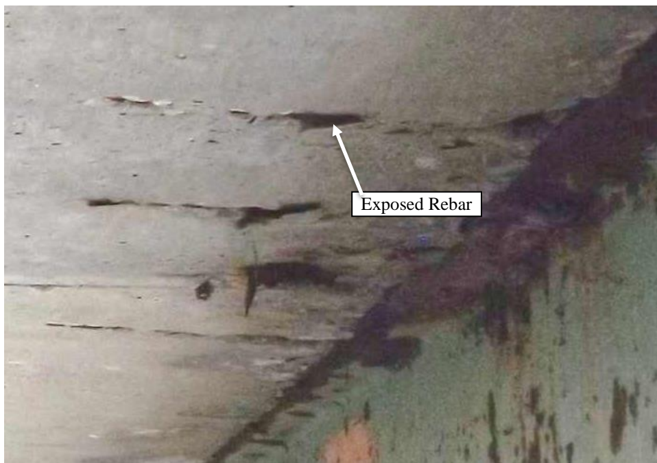
Figure 4.4 Concrete Deck Spalling with Exposed Rebar
