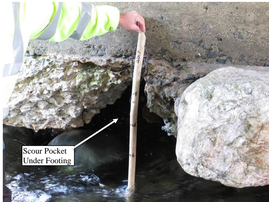
Figure 1.3 Scour Pocket at West Abutment
