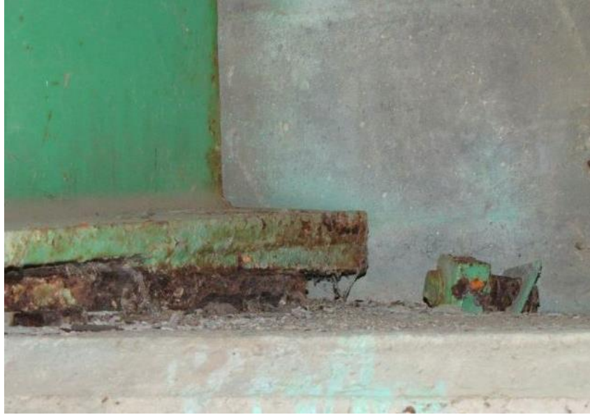
Figure 3.3 Typical Sheared Anchor Bolt
