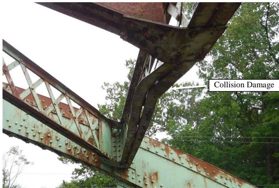
Figure 8.9 Collision Damage to West Portal
