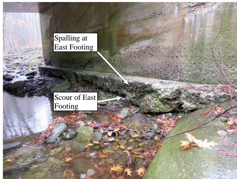
Figure 1.5 Scour and Spalling Along the East Footing
