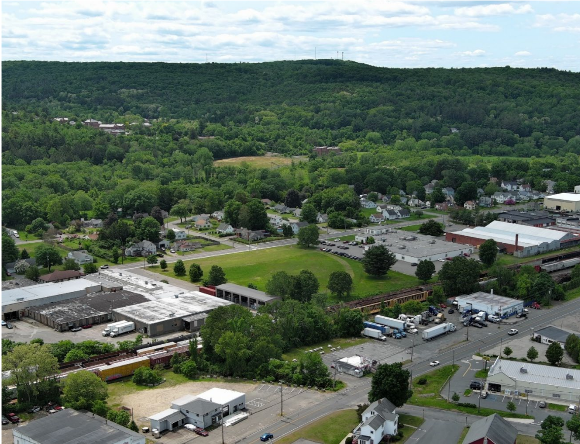
A southwesterly view towards the preferred station site at 1199 South Main Street.
