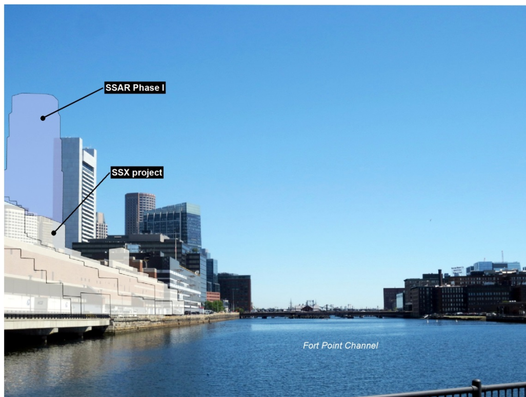
Figure 10—View of South Station site at Fort Point Channel looking north from Gillette – Alternative 2
