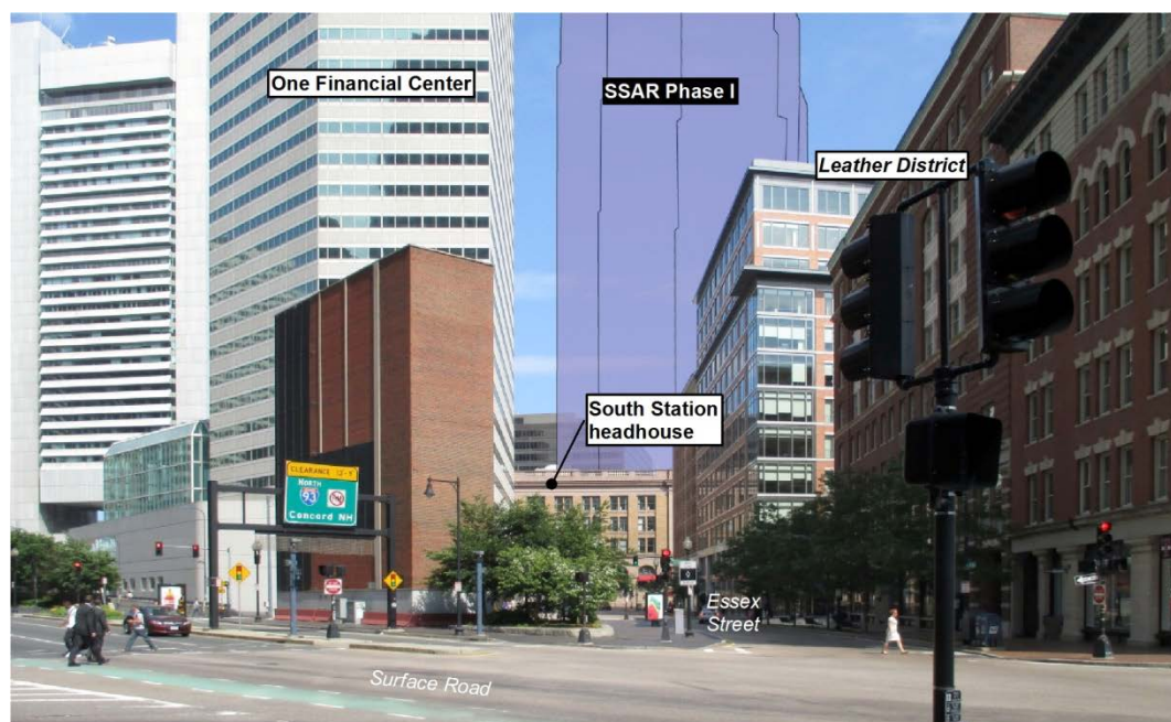
Figure 5—View of South Station site looking southeast along Essex Street from the Surface Artery – No Build and Build Alternatives
