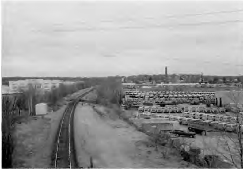
Readville Carshops, Industrial Drive: Overview
