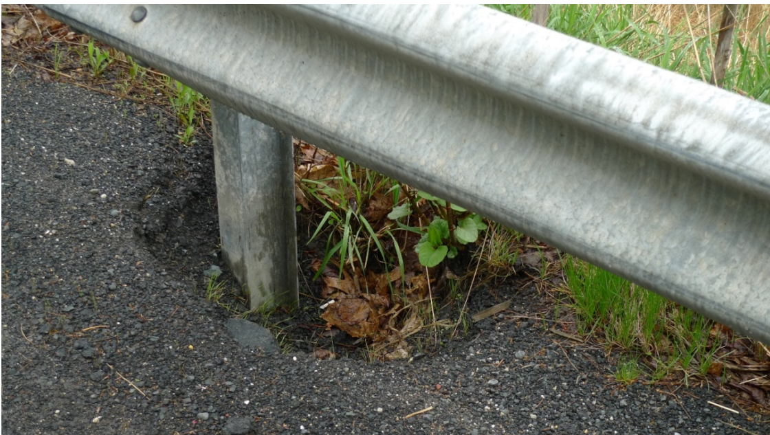
Figure 3.13: Conway erosion around guardrail footing
