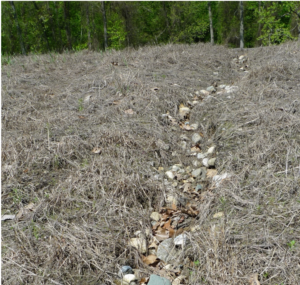
Figure 3.9: Deerfield rill erosion downslope from berm cut, May 23, 2019
