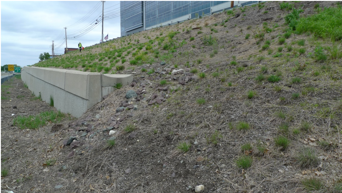
Figure 3.19: Erosion at south end of Waltham retaining wall, May 23, 2019
