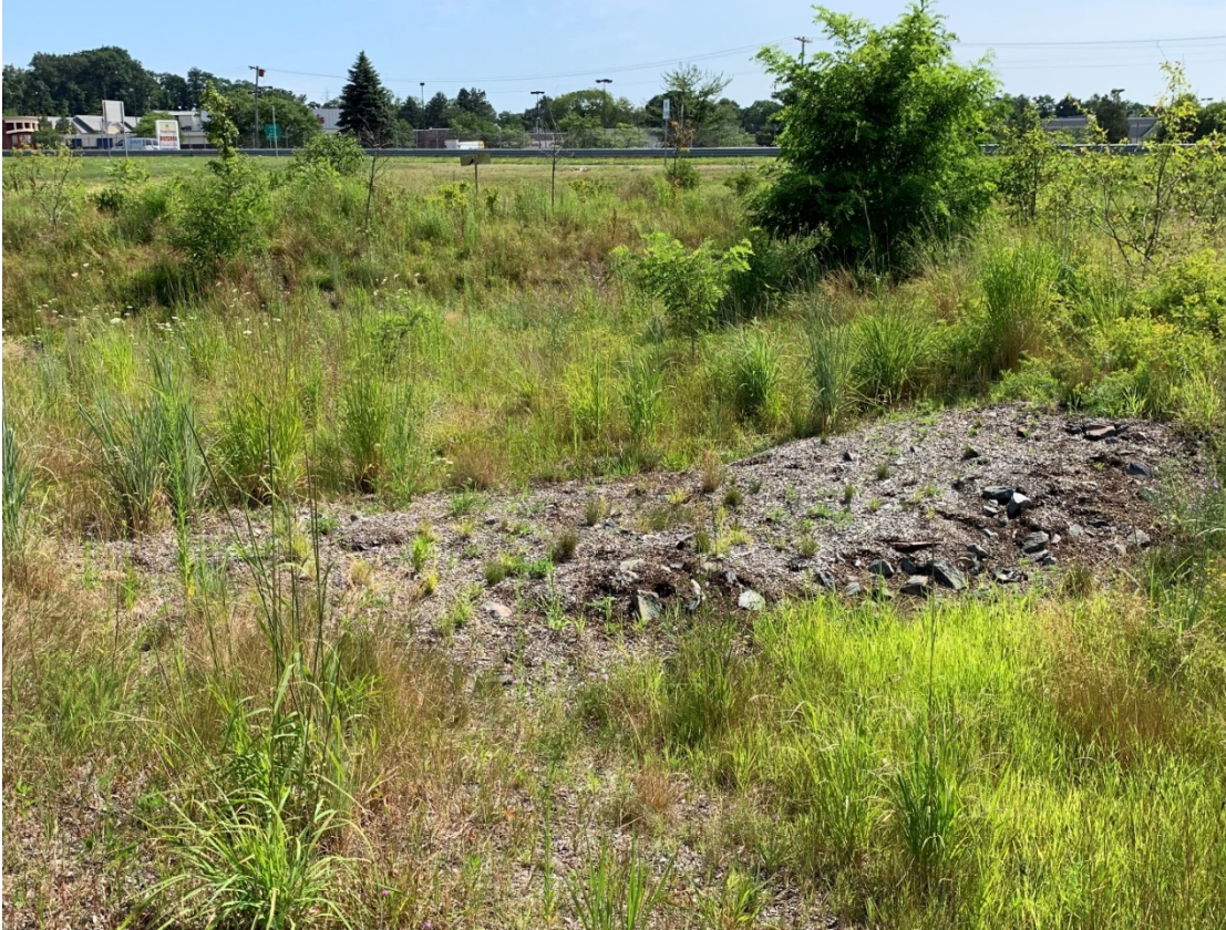
Figure 3.25: Danvers sparsely vegetated rip-rap berm, Aug. 6, 2019
