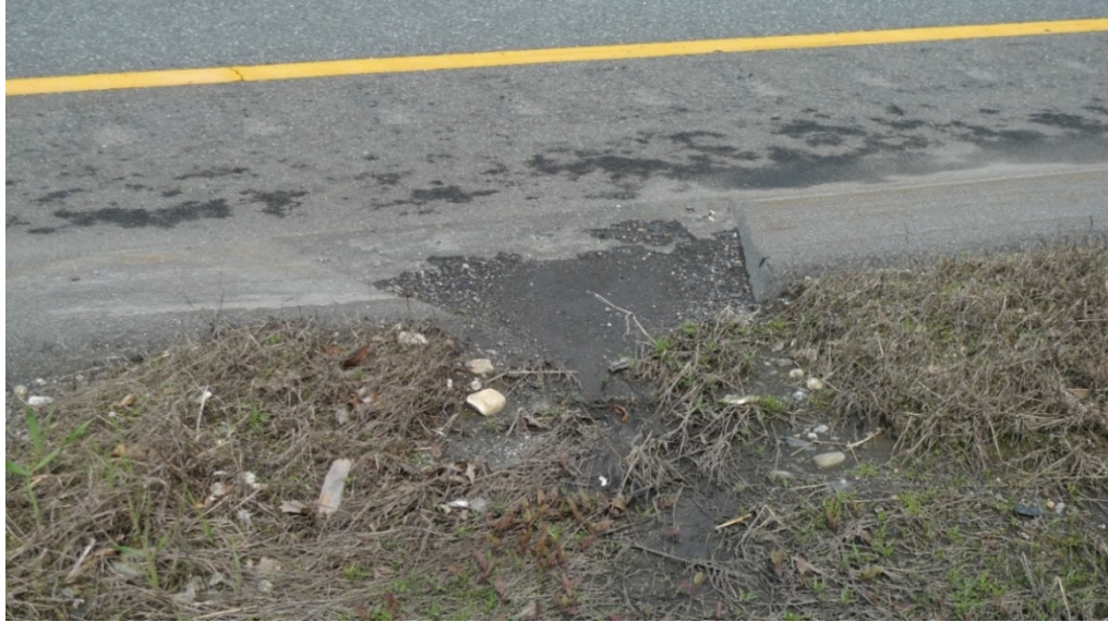
Figure 3.8: Deerfield Cape Cod berm relief cuts, May 23, 2019
