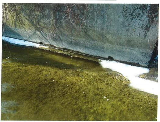
Photo 3: Typical retaining wall with exposed footing and failed weep pipes, northwest shown.
