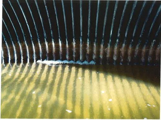
Photo 4: Typical condition of the pipe with rusting near and below the waterline, west shown.
