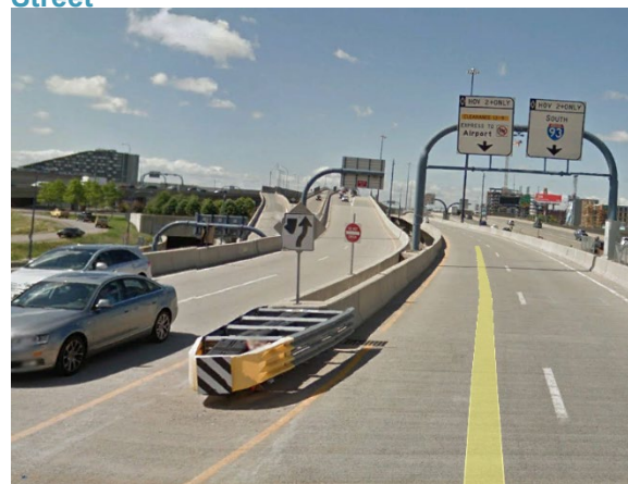
Figure 5 - I-93 SB HOV Lane at Kneeland Street
