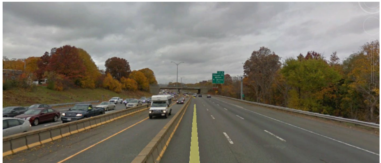
Figure 7 - Southeast Expressway HOV Zipper Barrier Deployed
