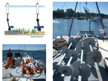
Figure 3. clockwise from left: diagram of a conservation mooring; helical anchors; conservation mooring (helical anchor and flexible rode) ready for installation in Manchester Harbor.
