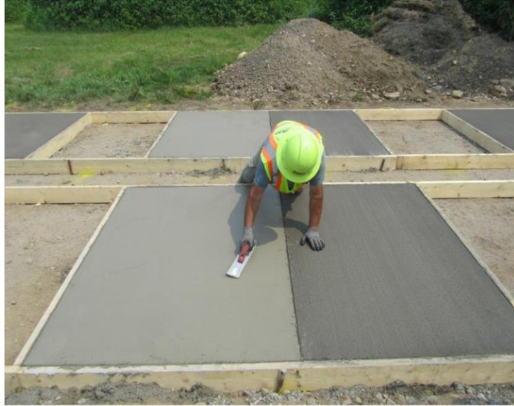
**Figure 2.2 Worker trowels sidewalk panel following MassDOT specifications**
