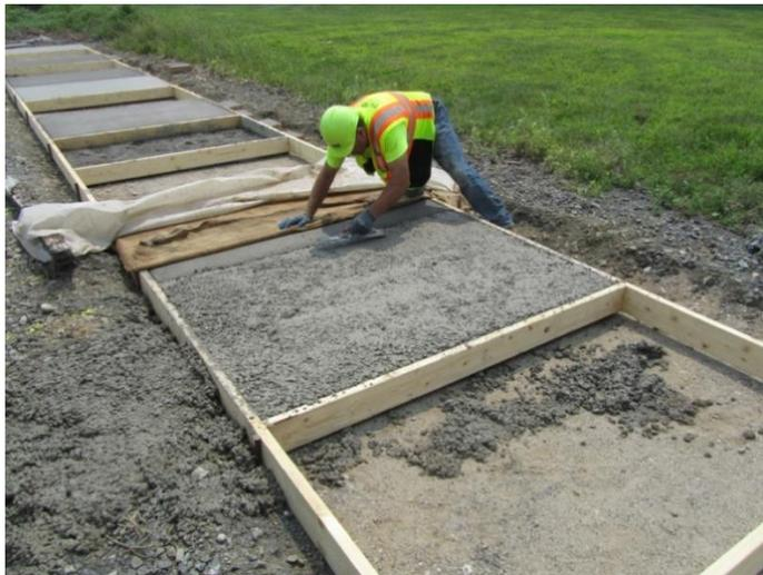
**Figure 5.5 Worker uses trowel on concrete panel**
