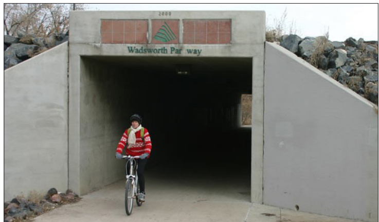
An example of a bike path through a box culvert.
