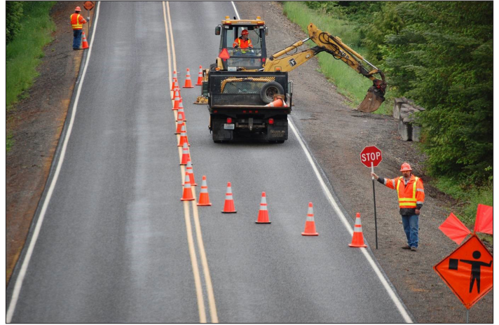
Temporary traffic control aims to move road users safely through or around work zones.
