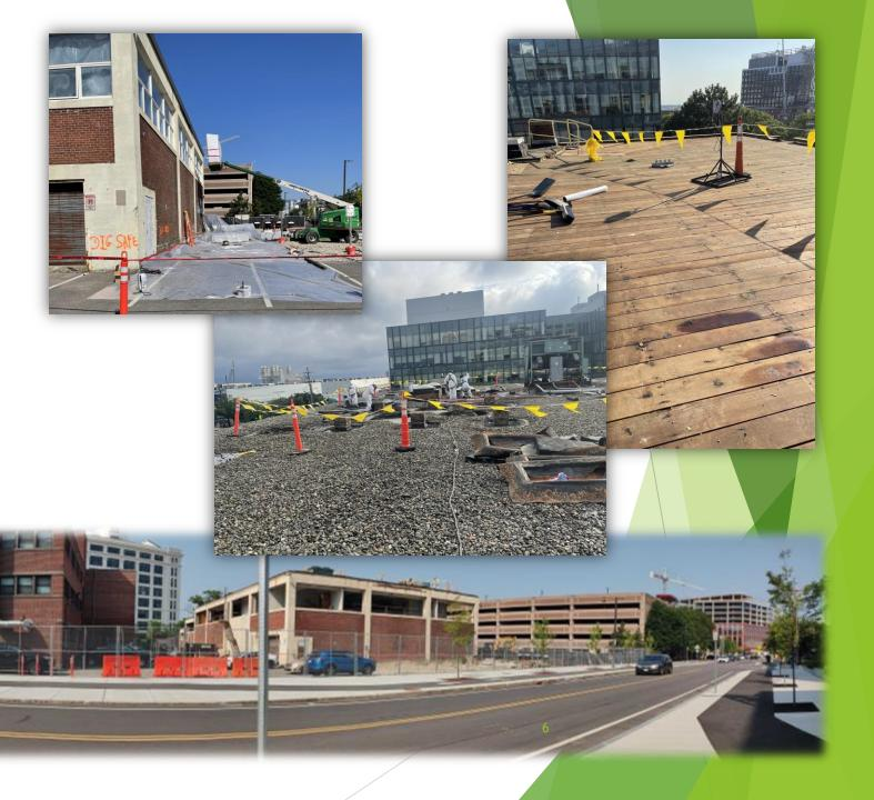
We had sequenced our work so that all asbestos abatement and an adjacent concrete structure had been demolished, leaving a clean slab for processing and stockpiling the 22 Drydock building material components. In a very systematic manner, we separate and remove building components to reveal the timbers to be harvested.
