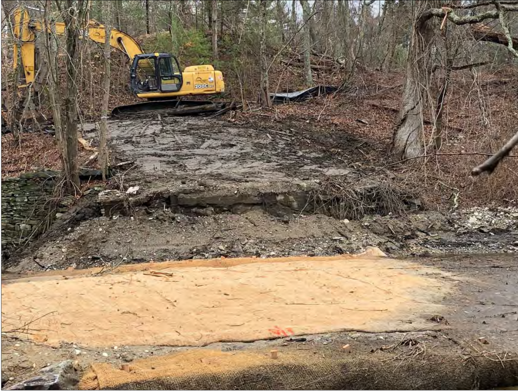
Figure 17. Removal of timber matting following completion of dam removal and river restoration machine work, view southeast.
