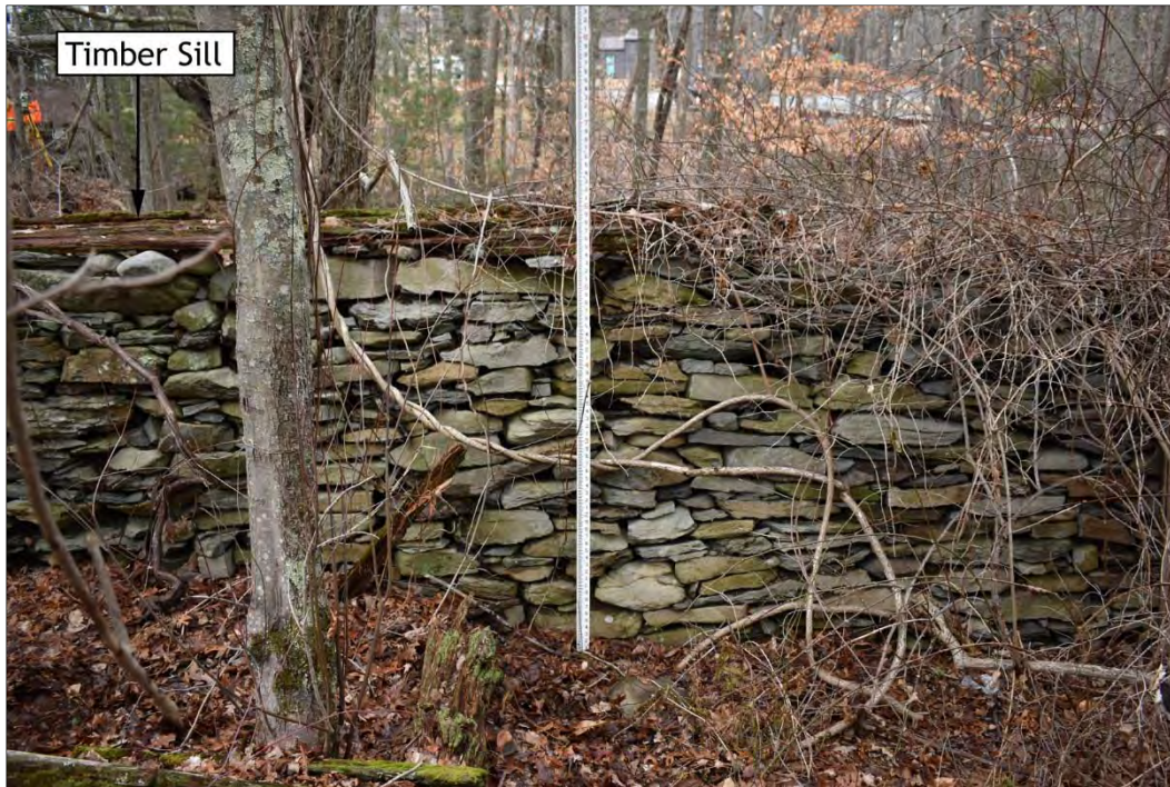
Figure 3. Dry-laid fieldstone foundation wall with timber sill east of dam, view northwest.
