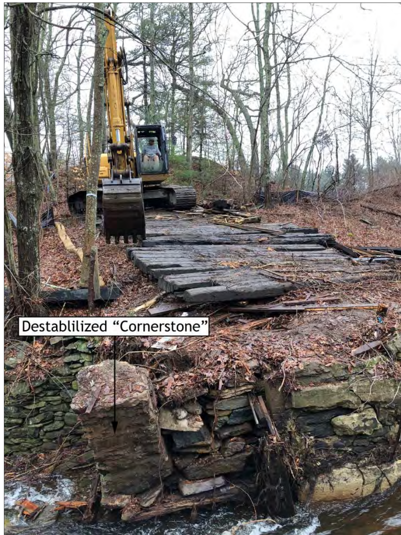
Figure 32. Destabilized corner stones of mill foundation in relation to timber matting and dam removal access road extension to east channel, view west.
