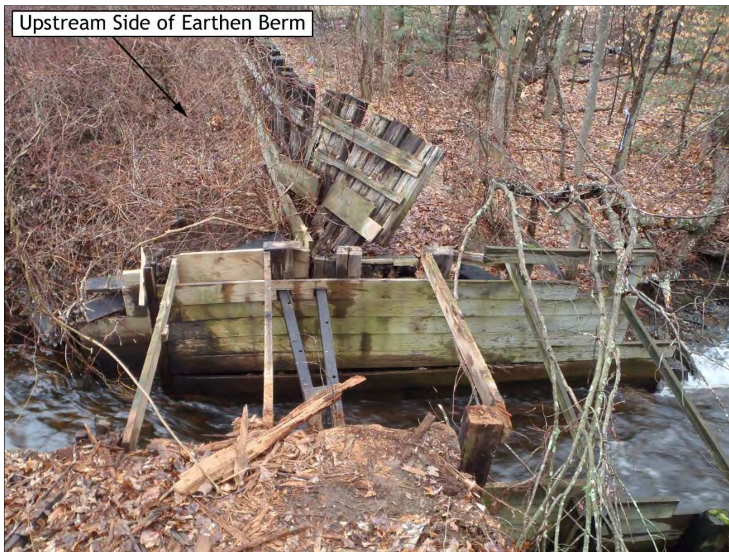
Figure 30. Removal of modern wood decking and boards lining the east channel through spillway section, with earthen berm dam component in the background, view northwest.
