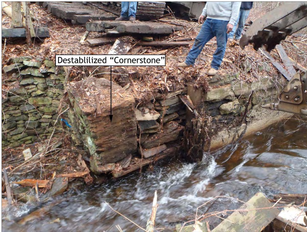
Figure 31. Destabilized corner stones of mill foundation at spillway in east channel, view southeast.
