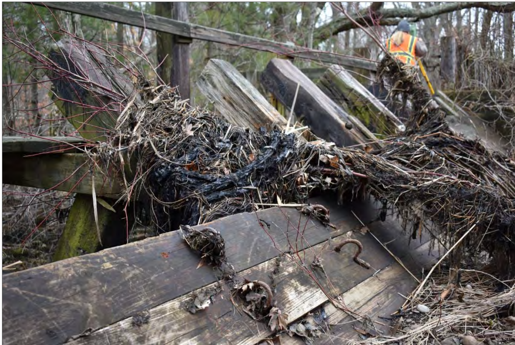
Figure 25. Upstream face of dam with removable wood planking, view southeast.
