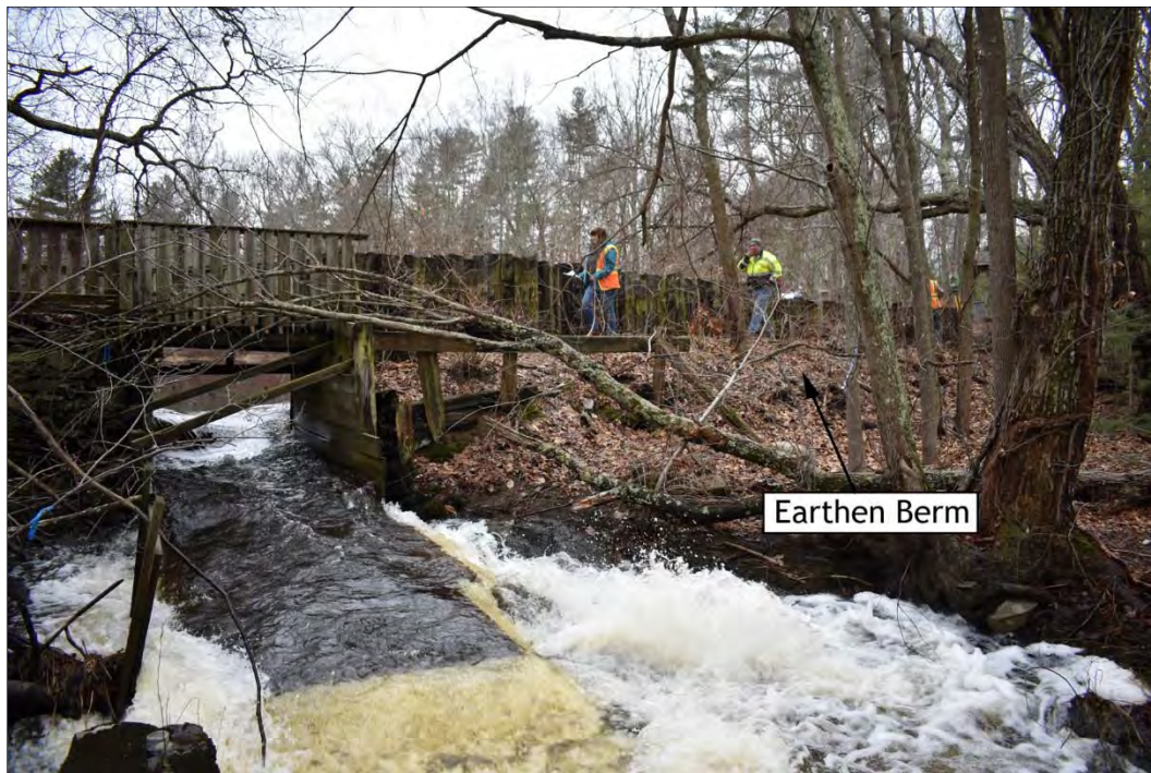
Figure 19. Earthen berm component of Barstow's Pond Dam structure, view southwest.
