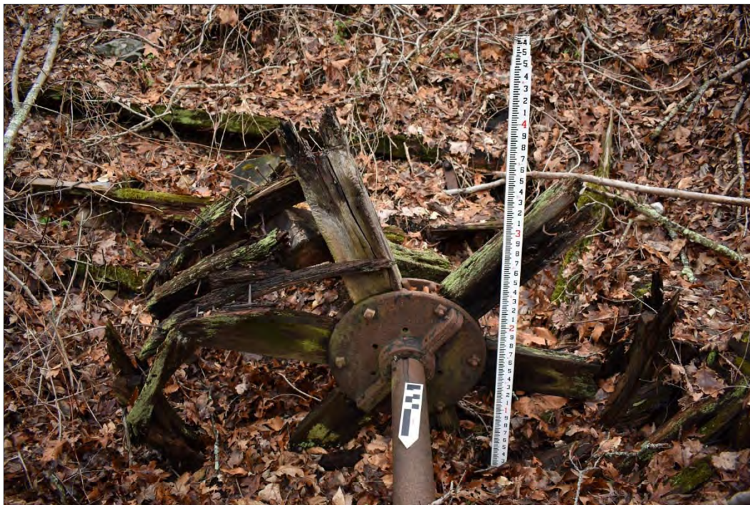
Figure 6. Detail of wooden water wheel remains inside cellar hole of mill building, view northwest.
