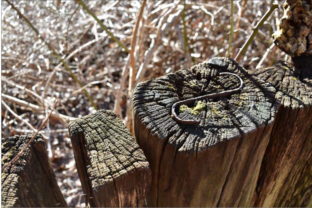
Figure 21. Iron S-shaped pin embedded in short end of vertical wood timbers in earthen berm component of the dam.
