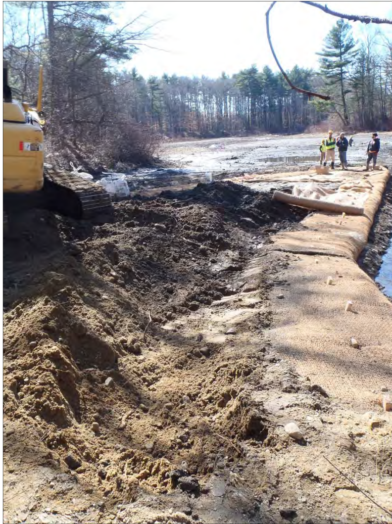
Figure 43. Excavation of the earthen dam component and west channel bank treatment, view southwest.
