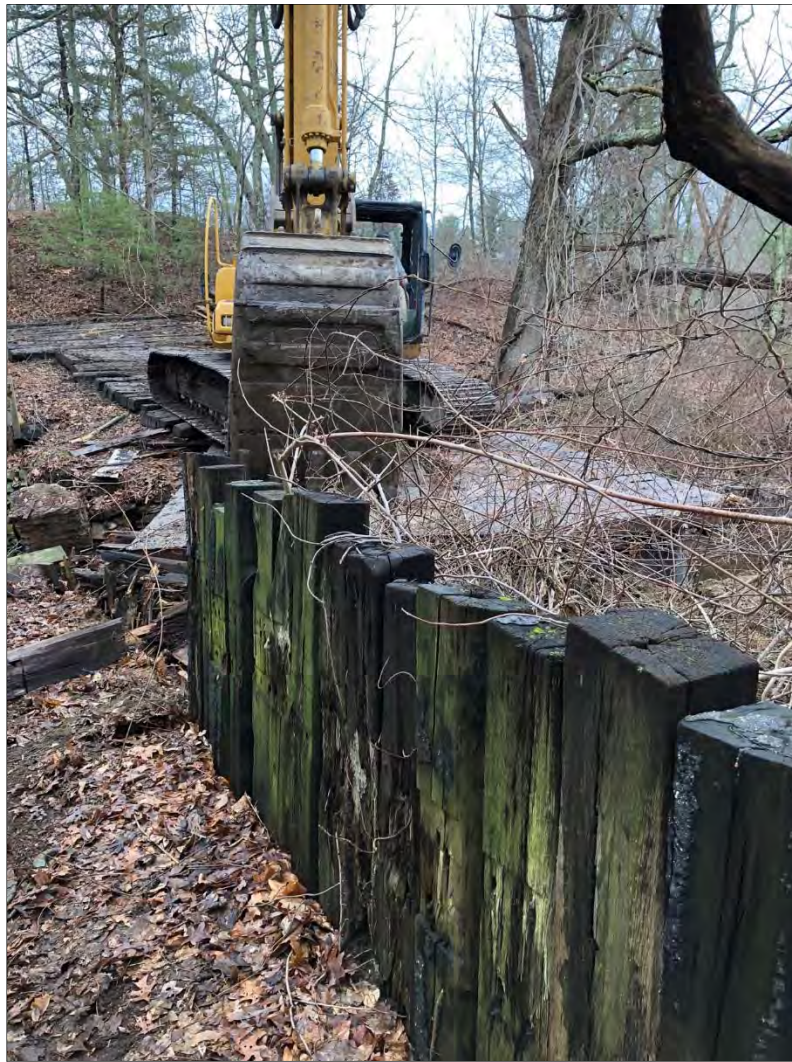
Figure 20. Vertical wood timbers along upstream side of earthen berm component of the dam, view southeast.
