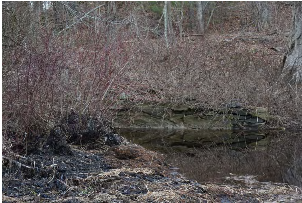
Figure 12. Mill foundation wall sections composed of parged concrete over fieldstone foundation wall not documented during 2013 intensive survey, view south: a) wall section under former wood plank deck; and b) wall section lining upstream eastern channel (spillway) at west side of former wood plank deck.
