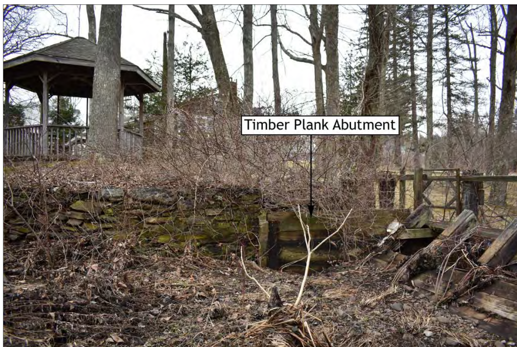
Figure 26. Western wood abutment of timber dam section and dry-laid stone retaining wall, view northwest.
