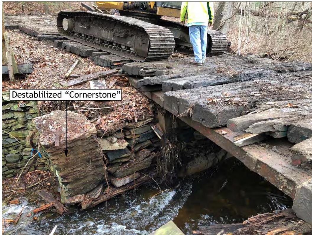
Figure 34. Realigned timber mats and construction access across east channel (spillway), view southeast.
