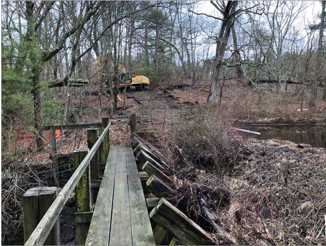
Figure 27. Vertical wood posts and wood plank deck over top of timber dam section, view southeast.
