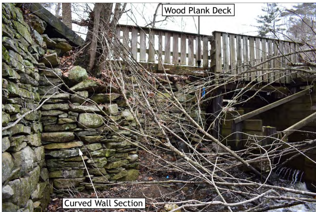
Figure 11. Curved dry-laid fieldstone foundation wall section not documented during 2013 survey, view southwest.
