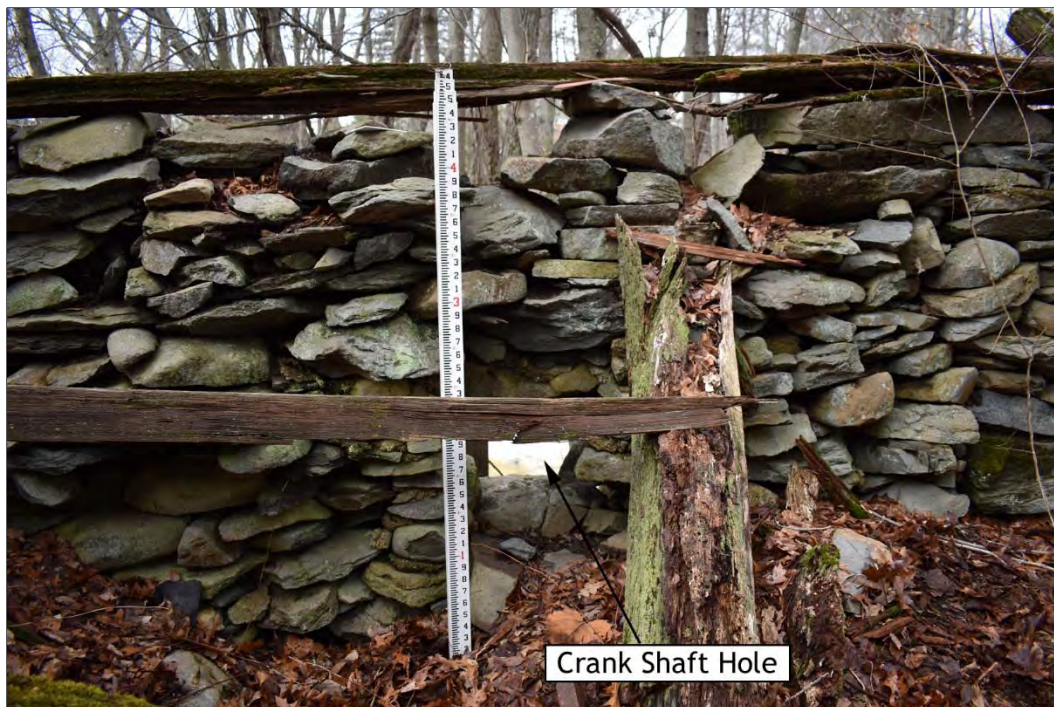
Figure 9. Detail of square hole in foundation wall between two wheel pits, view northwest.
