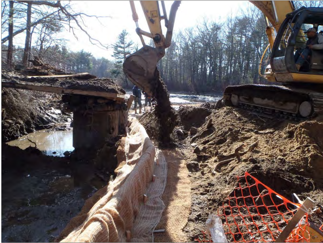
Figure 44. Excavation of earthen dam component and eastern channel bank treatment, view southwest.
