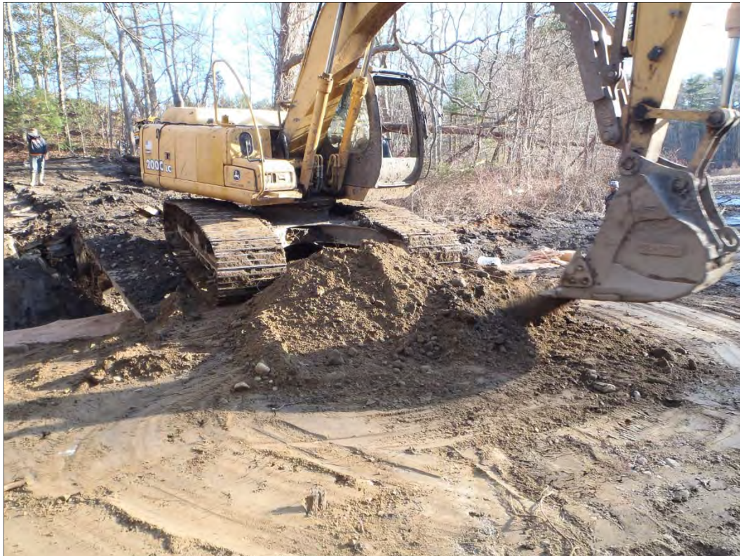
Figure 42. Excavation of west portion of earthen dam component to construction grade, view southeast.
