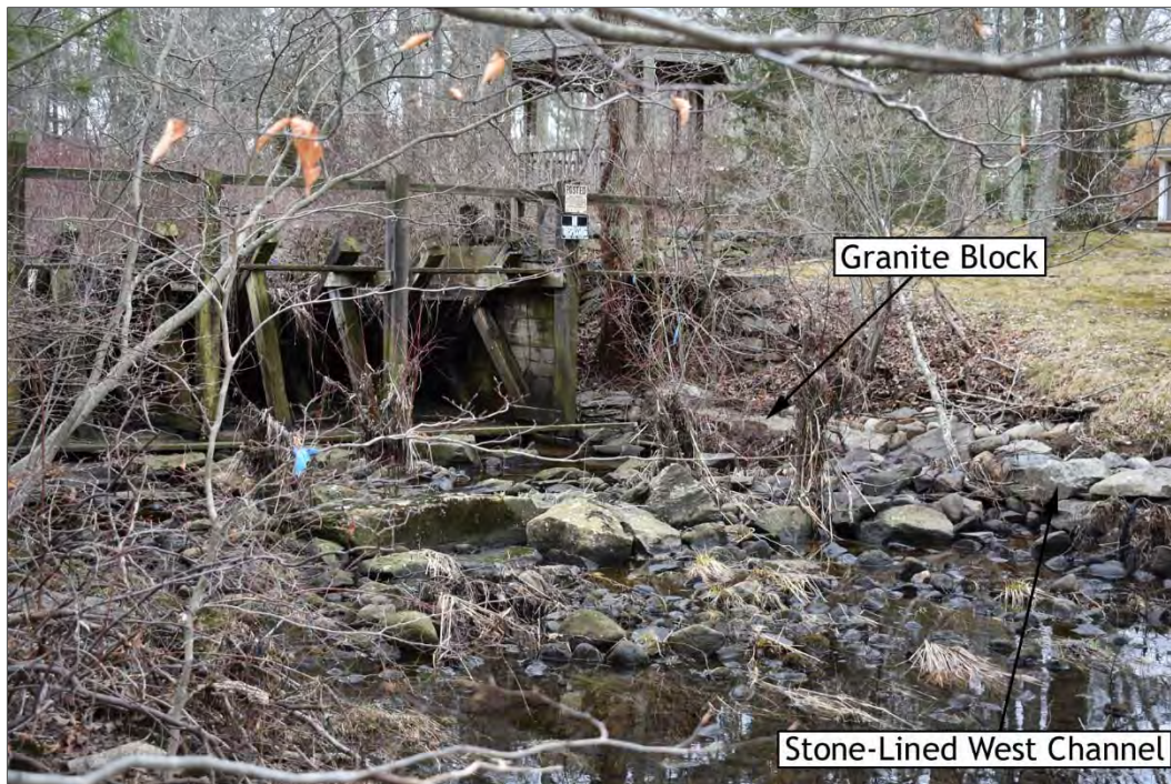
Figure 28. Timber dam section, cobble river bed, and stone-lined west channel, view southwest.
