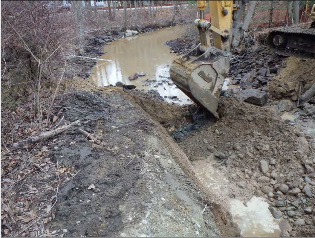
Figure 41. Reconstruction of west channel and riverbank in the area of former timber dam component, view northeast.
