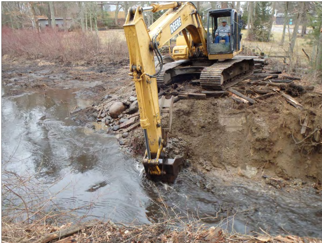
Figure 39. Contractor excavations in east end of earthen dam at east channel, view northwest.
