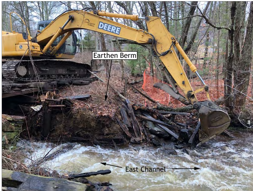
Figure 36. Contractor excavations in east channel (spillway) to facilitate upstream pond drainage, view east).
