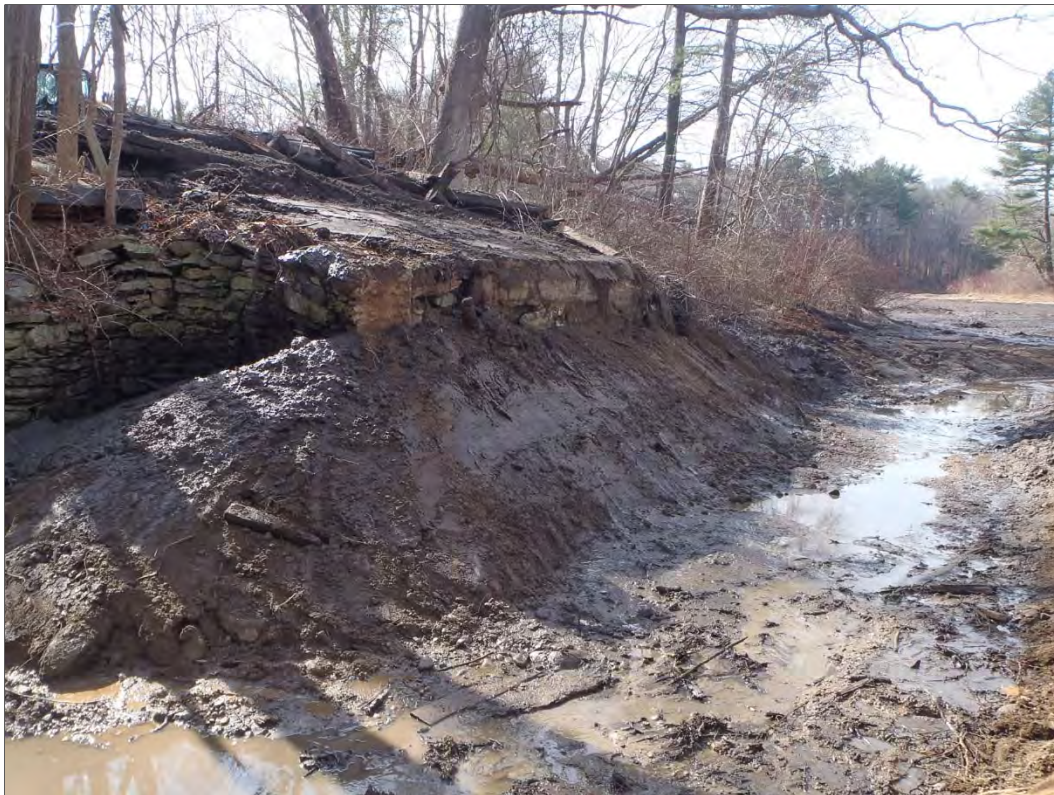
Figure 35. Finished sloped grade of east side of realigned eastern channel along mill foundation fieldstone wall, view southwest.
