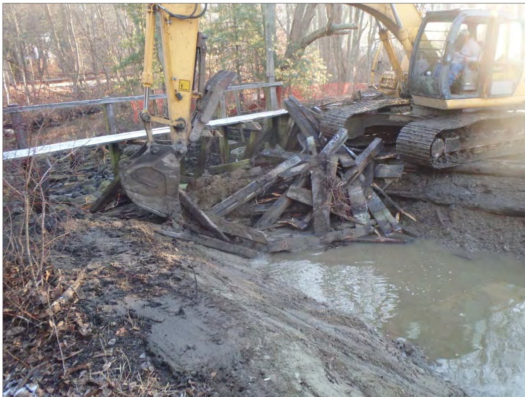
Figure 40. Removal of timber dam from the east on remaining upstream portion of earthen dam fill, view east.
