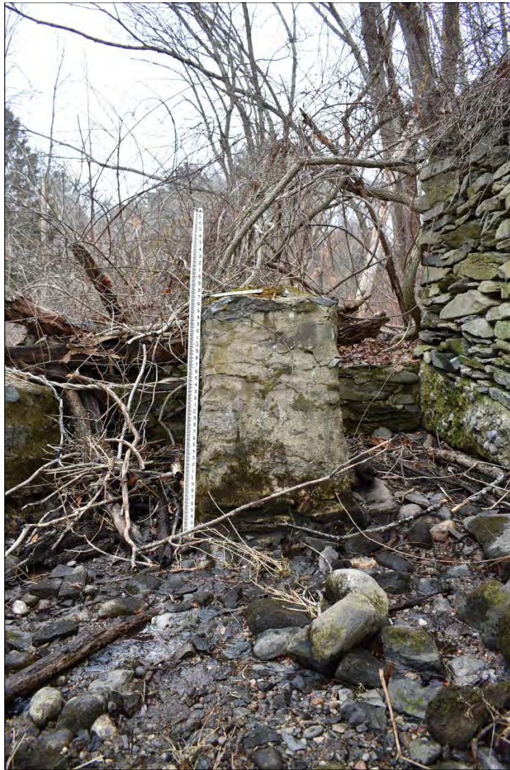
Figure 7. Mortared fieldstone pier for western (exterior) water wheel, view northeast.
