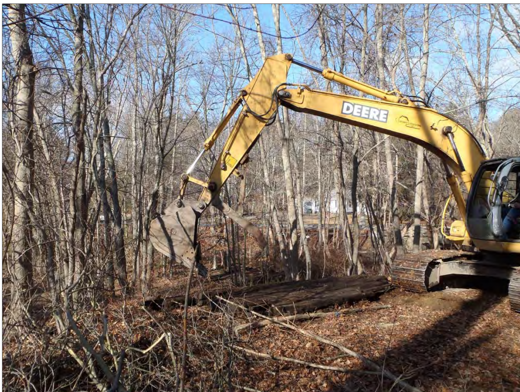
Figure 16. Installation of timber matting on west side of the east channel (spillway), view northwest.
