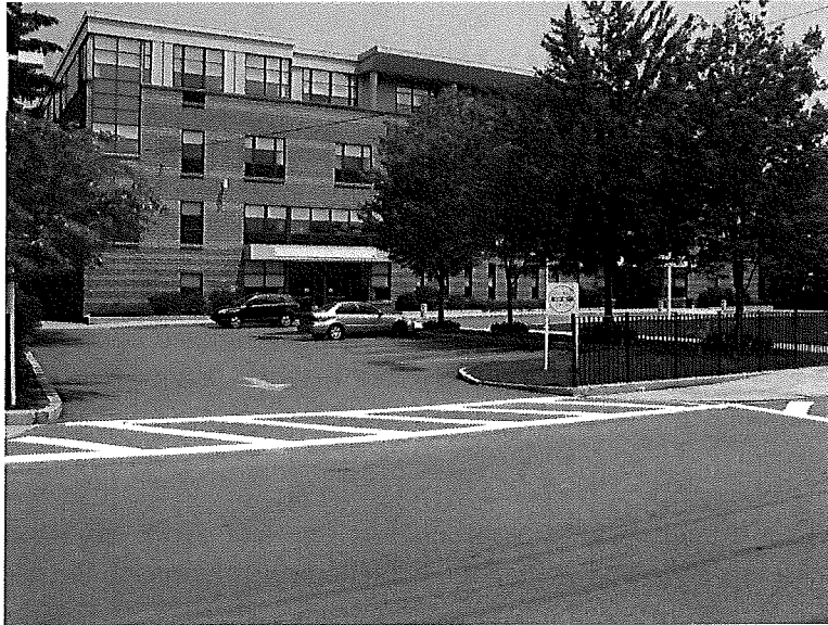
Figure 4 – Crosswalk markings located in front of the school
