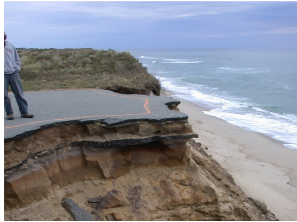
Photograph 2.17. Destabilized coastal bank. The construction of, use of, and stormwater runoff from this pavement has contributed to erosion and destabilization of the top and face of the coastal bank, yet due to its significant height, this bank still acts as a vertical buffer. This bank also provides sediment to the adjacent beach.
