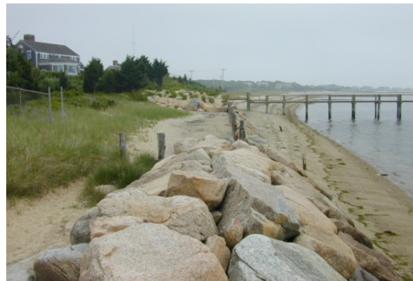
Photograph 1.9. Coastal dune with coastal engineering structures. Foreground: coastal dune landward of rock revetment. Background: coastal dune and beach landward of a deteriorated bulkhead.
