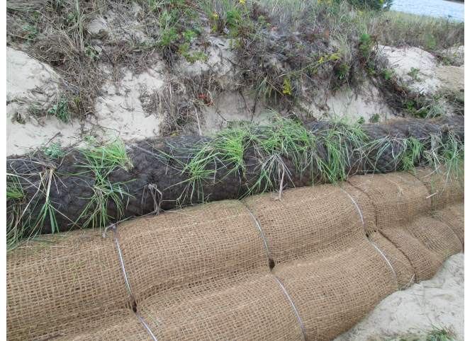
Photograph 3.1. Coconut fiber rolls used to stabilize the toe of a coastal bank. These rolls (some of which were wrapped in natural fiber blankets) were later covered with sand and planted .
