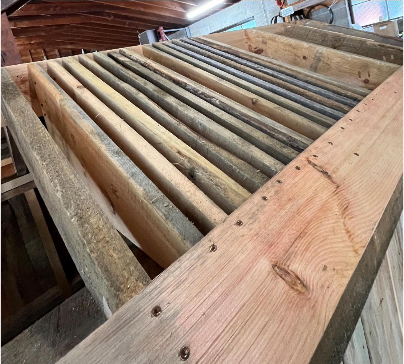
2 Baffles installed between roof rafters of "bat shed" to encourage roosting; structure to replace house scheduled for demolition, baffles crafted in accordance with recommendations by MassWildlife
