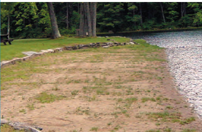
At Mauserts Pond (Clarksburg State Park), grass encroaching on the beach area was tilled and re-surfaced with three inches of beach sand.
