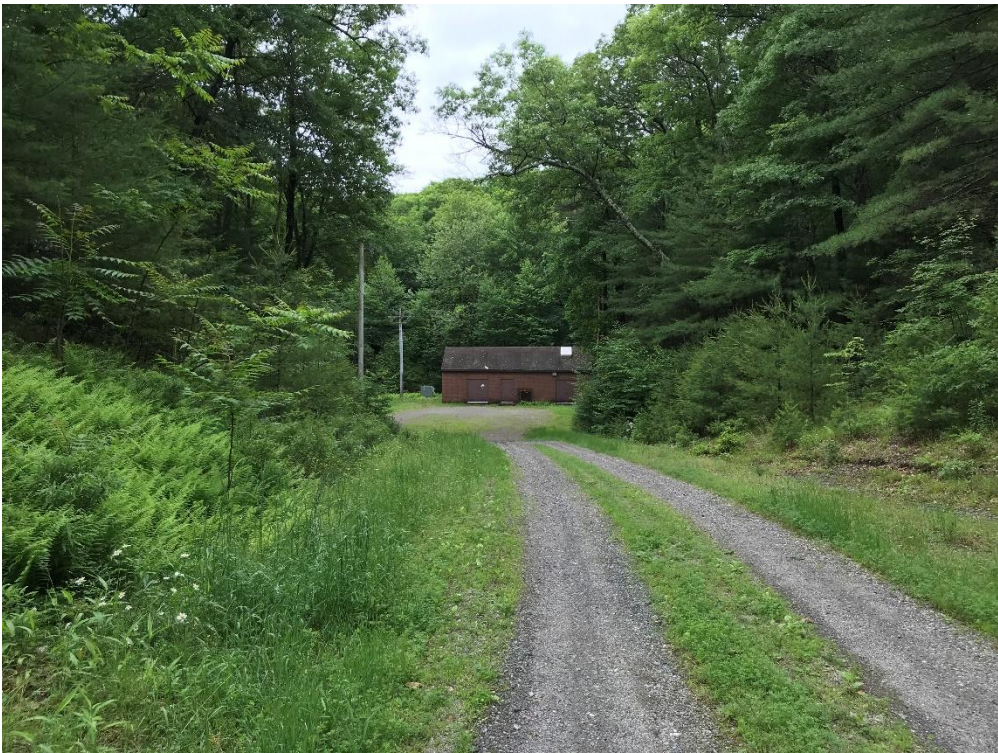
C. Boylston Water Dept building
