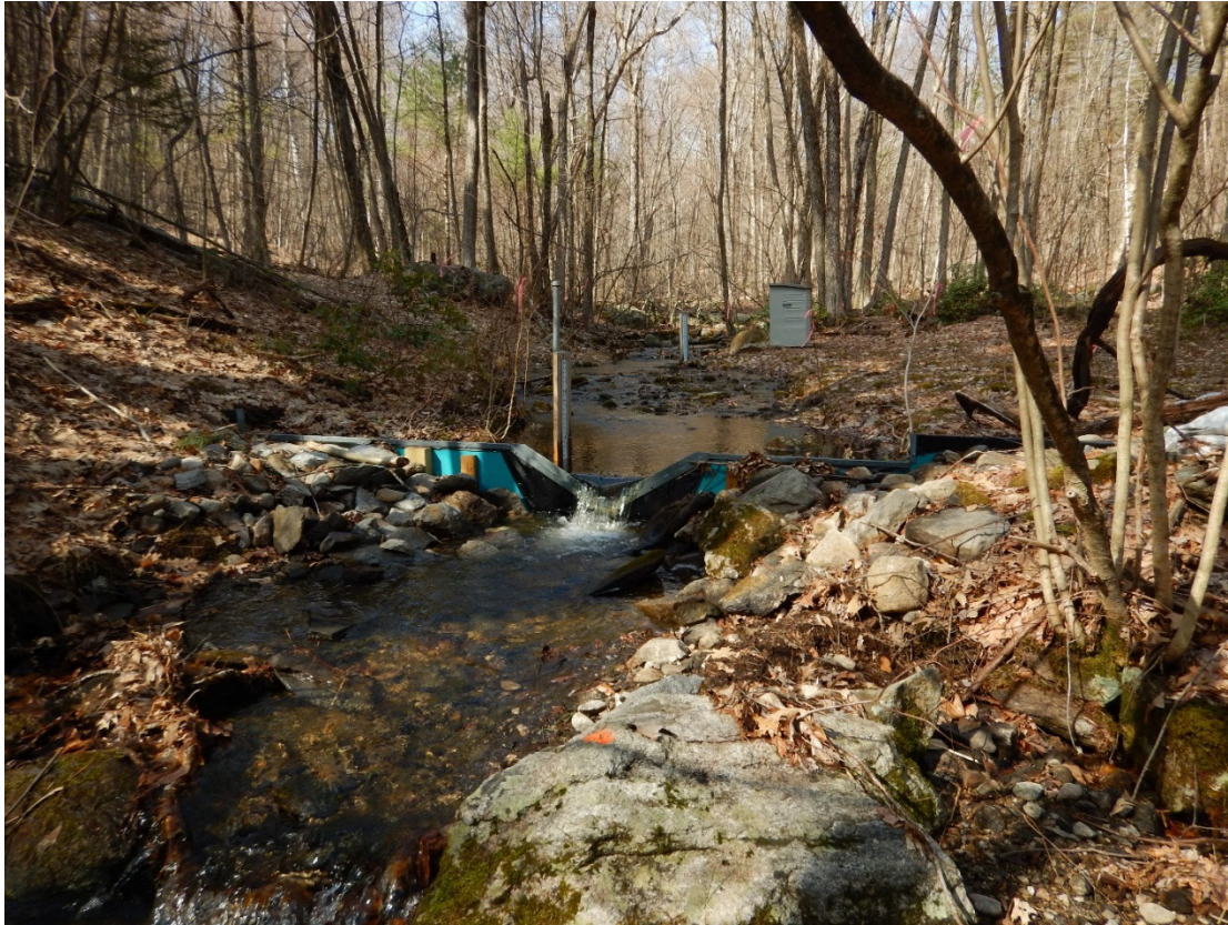
A. Weir that was installed in order to monitor stream flow.
