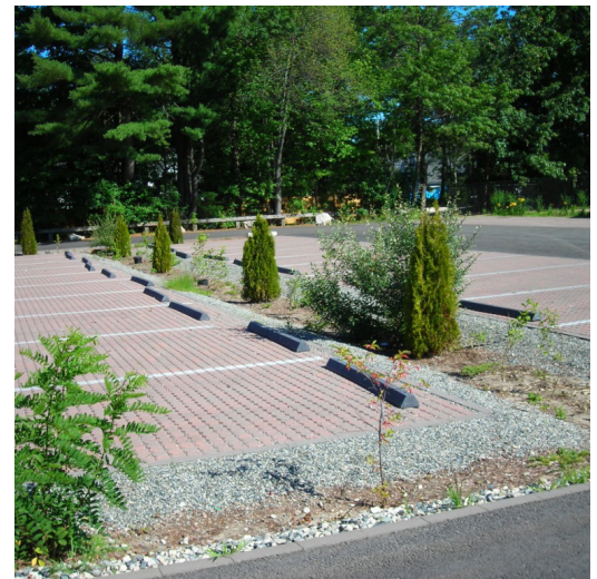
Image 6. Example installation of permeable pavers, permeable pavement, and a bioswale at Silver Lake Beach in Wilmington, MA. (Source: Sara Cohen, DCR Office of Water Resources)
