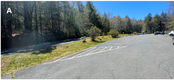
Image 2. Stormwater runoff from the large parking lot (Image 2A) flows rapidly down the steep slope towards the beach, causing beach scouring and erosion. The stairway connection between the parking lot and the beach shoreline (Image 2B) illustrates the sharp grade. Bioswales along the edge of the parking lot and road will help to alleviate these impacts.
