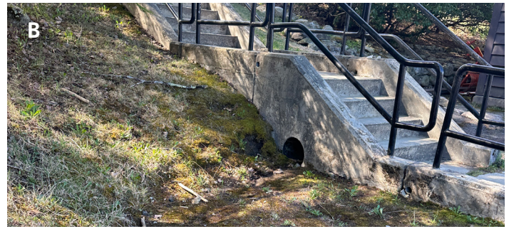
Image 2. Stormwater runoff from the large parking lot (Image 2A) flows rapidly down the steep slope towards the beach, causing beach scouring and erosion. The stairway connection between the parking lot and the beach shoreline (Image 2B) illustrates the sharp grade. Bioswales along the edge of the parking lot and road will help to alleviate these impacts.
