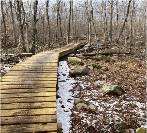
Boardwalks and puncheons allow users to visit resource areas without impacting the soil
