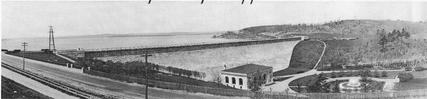
Wachusett Dam and Grounds, Clinton, MA, ca. 1919. The 40" x 8" original nitrate cellulose panoramic negative was found in a tube at the back of a storage closet in the Wachusett Dam Administration Building (above) in fall 1999 by an employee of the MDC Division of Watershed Management, Wachusett Section. The Northeast Document Conservation Center (Andover, MA) was contracted to make contact prints from this negative. The above image is a detail of a 50% reduction of the original negative, which is now archivally enclosed in buffered tissue paper and in a buffered tube. It will be transferred to the Massachusetts State Archives during the course of this project.
