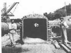
48-inch pipes through the Wachusett Dam, Sept. 6, 1902
