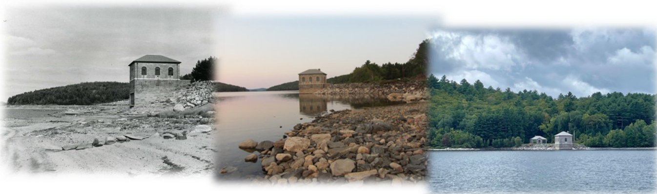
Quabbin Shaft 12 Intake at three different drought stages (from top left): 10/13/1966 – elevation 496 feet; 9/5/2016 – elevation 521 feet; 9/20/2022 – elevation 524.57 feet.
