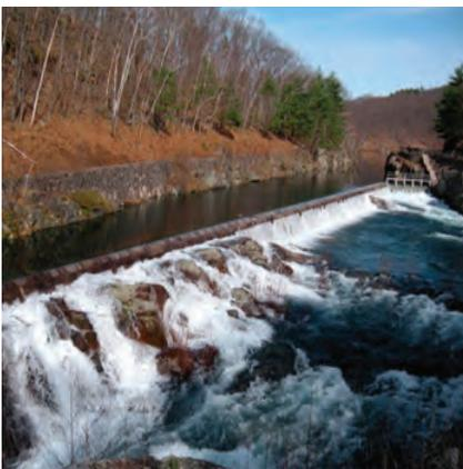
The Quabbin Reservoir's spillway releasing water over the top of the wall (used when the reservoir exceeds 100% capacity) and the lower spillway. The lower spillway enables water releases even when the reservoir is not completely full.
