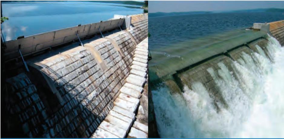
Wachusett crest gates, raised (at left) and lowered (right) allowing excess water to flow through the spillway and into the Nashua River
