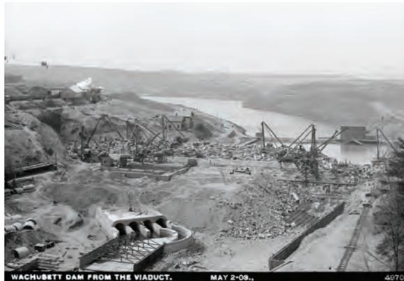
Center: Construction of the Wachusett Dam in May 1903 (top) shows the discharge pipes that will carry water from under the dam, through turbines, and down the Nashua River through a fountain. The base of the fountain can be seen below, along with significant progress on the dam in just five months. Right: The Quabbin Outlet works and channel under construction in 1940 (top) and completed in 1941 (below).
