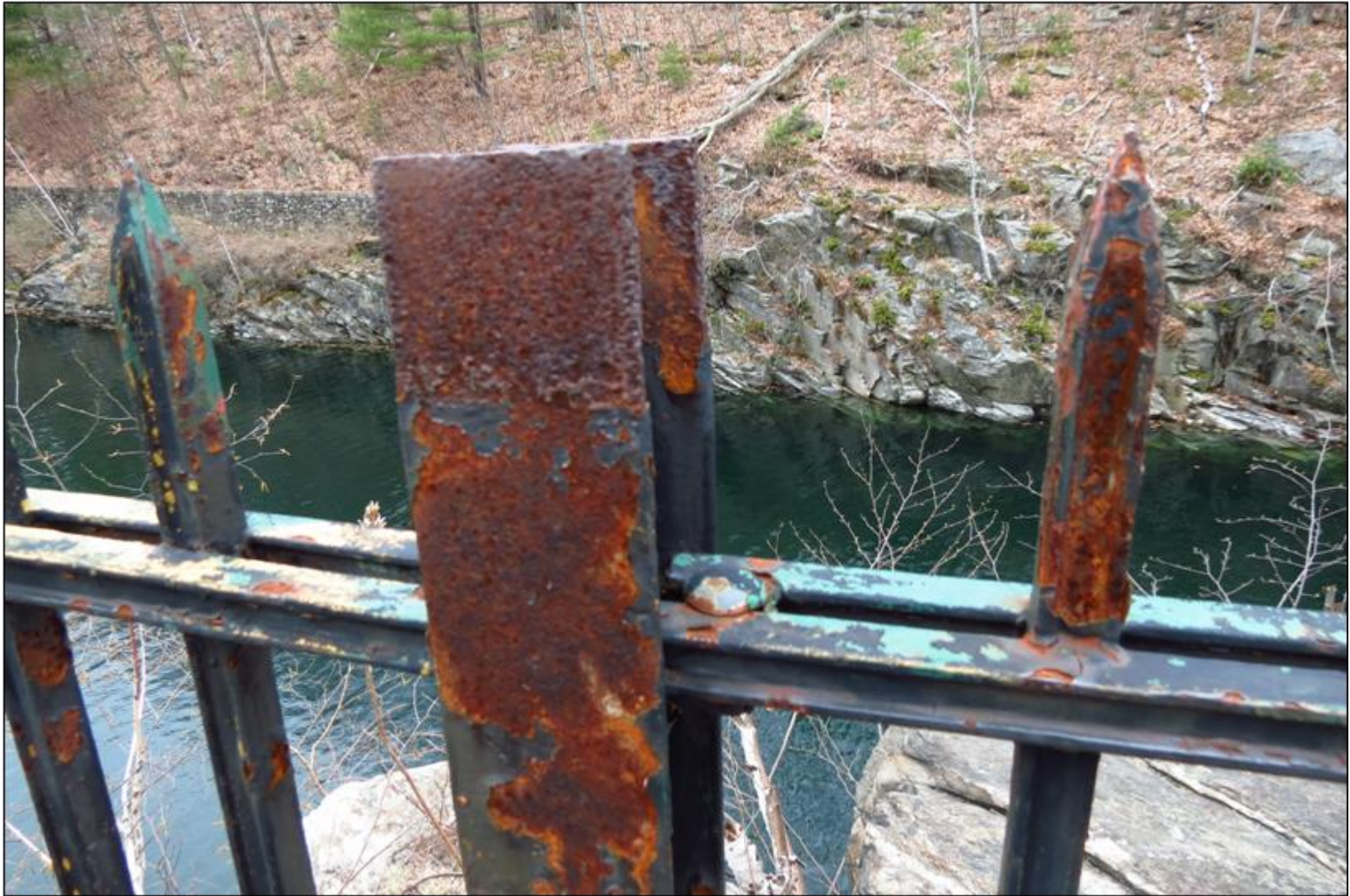
The top of the anchor post which is attached to fence sections on either side and sunk into the stone base below.
