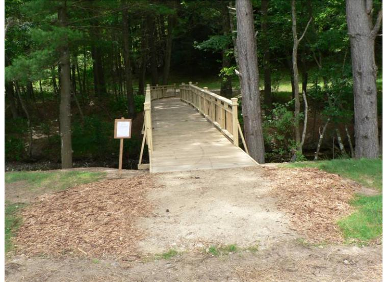
Top railings were added to meet code (above), and then finished off with balusters and caps (above right). Soil was added at either end to make the approach to the bridge level. Wood chips were also added for landscaping and to reduce erosion problems. The height of the bridge above the river allows unimpeded access for anglers who patrol this section of the river in search of trout (right).
