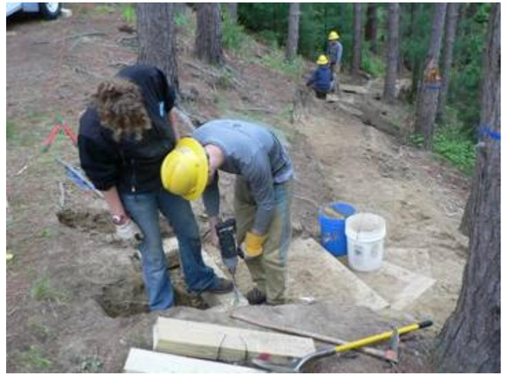
Steps along the steepest portion of the trail are cut into the bank, placed and secured (above). The upper terraces are put into place, leveled secured with pipe pins on the corners and stabilized from beneath with rocks and soil (below).
