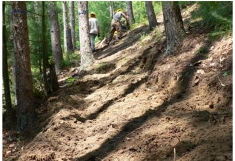
The new trail route is marked and cut (above), then roughed in (right). Terrace timbers are cut, then placed in trail before being secured with pipe posts and rocks (below). The trail takes shape (below right).
