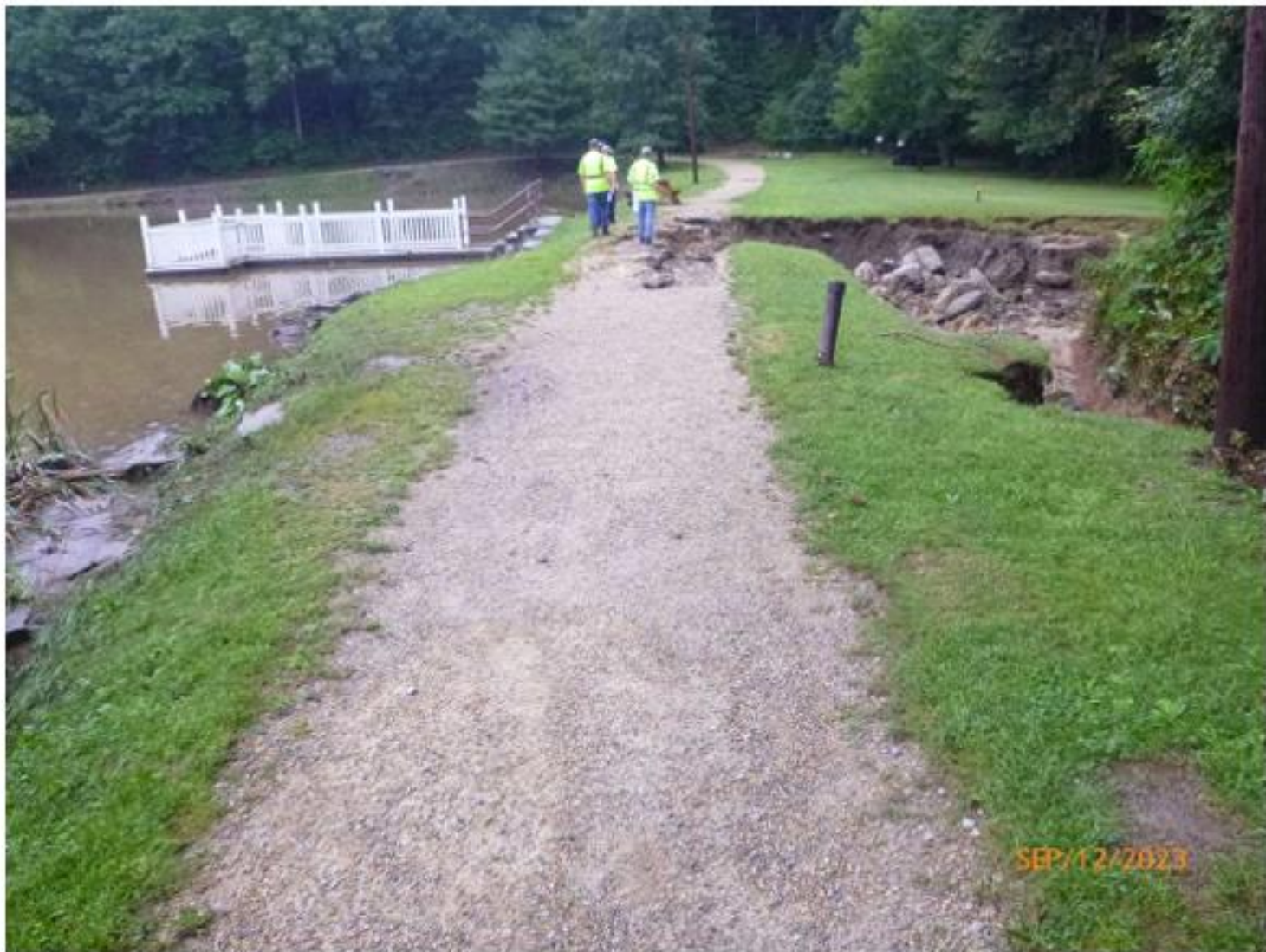
Photo 6 –Overview of embankment crest looking left. Note downstream slope failure due to overtopping
