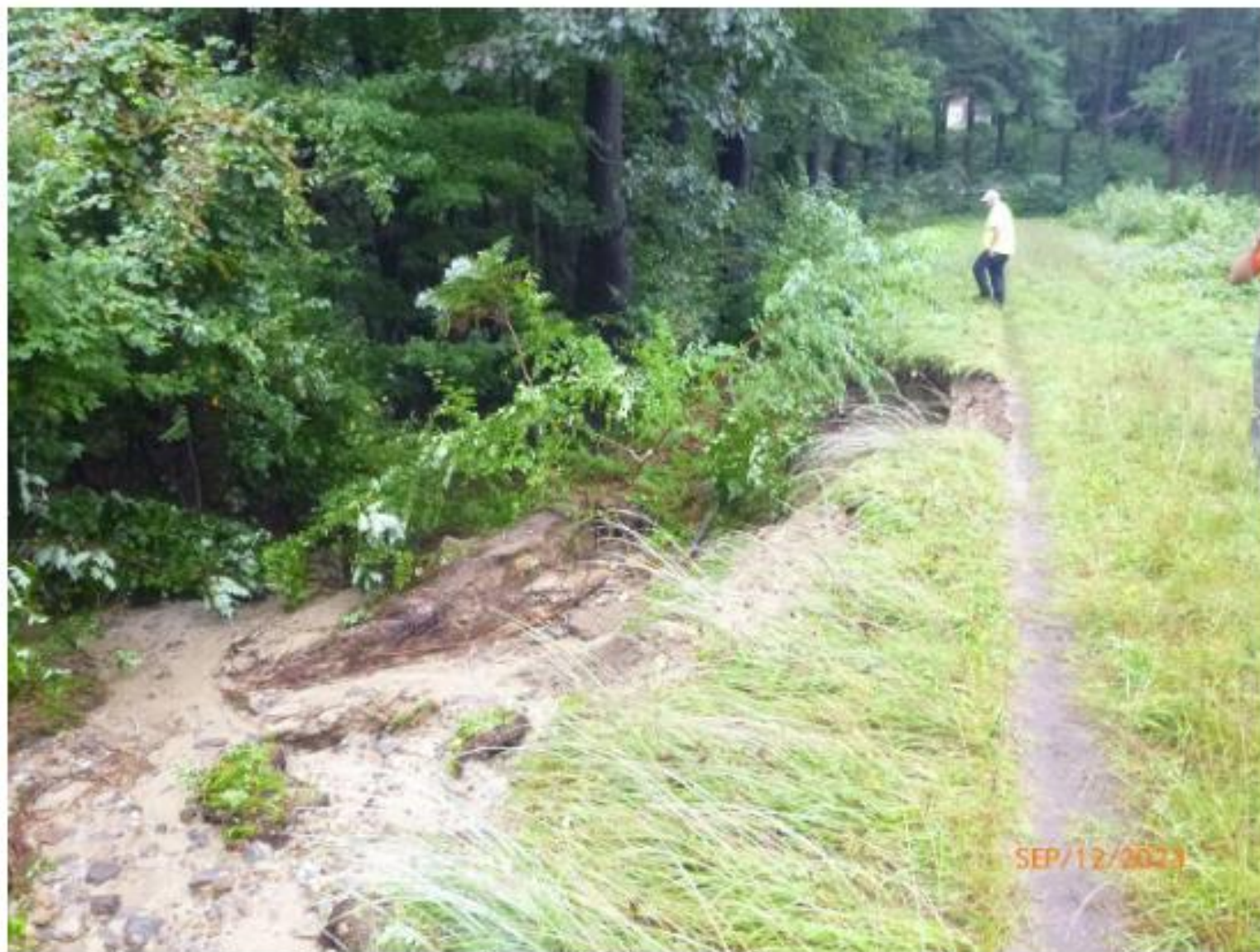
Photo 6 – Alternate view of slope failure due to overtopping
