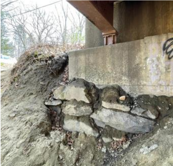
Erosion of the abutment footings
