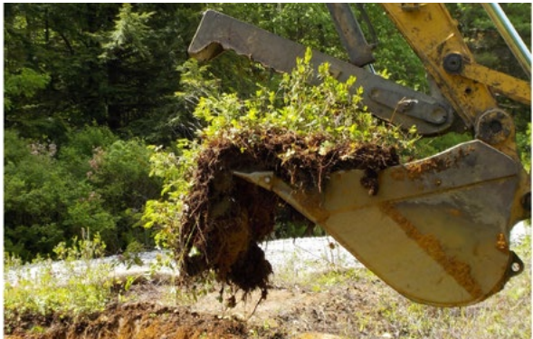
Innovative practices like translocating large blocks of soil with their established plants allows for more rapid wetland replication while preserving more of the beneficial soil function when compared with traditional practices. (G.Davies, BSC Group)
