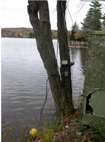
Lake Ashmere: Phone Lines Not in Compliance with State and Local Building Codes Running through Trees and Underwater
