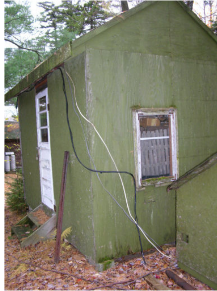
Lake Ashmere: Wiring Not in Compliance With State and Local Codes
