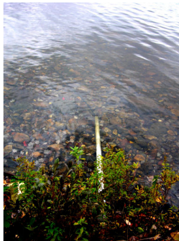
Lake Ashmere: Phone Lines Not in Compliance with State and Local Building Codes Running through Trees and Underwater
