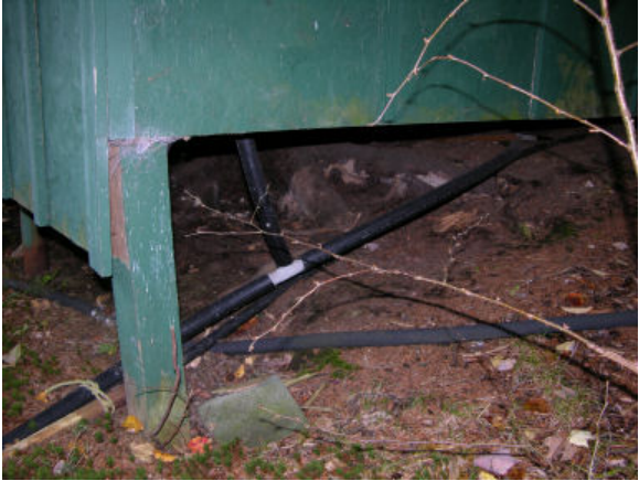
Lake Ashmere: Plumbing Not in Compliance with State and Local Codes
