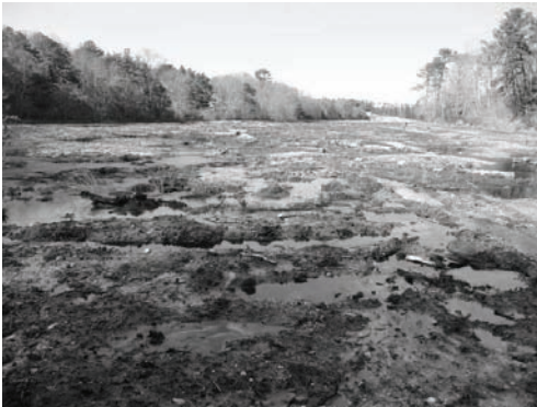
April 2010, Immediately following construction
