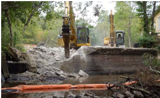
Contractors begin dismantling the Wapping Road Dam in September 2011.
