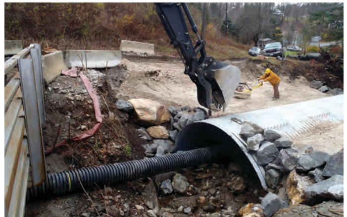
Contractors installing a wildlife-friendly culvert on Thunder Brook in Cheshire
