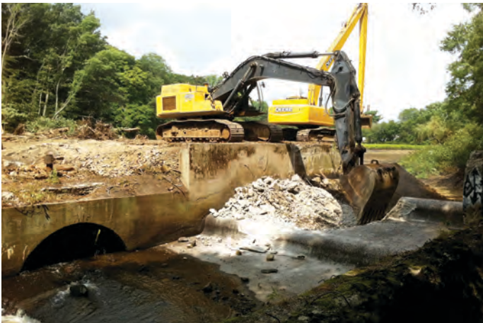
Machines begin to remove the Hopewell Mills Dam in Taunton, and then...
