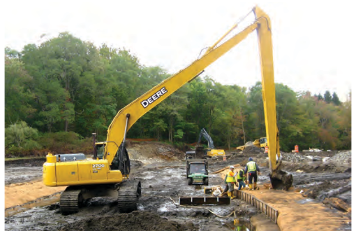
... rebuilding a stream channel through the former impoundment.
