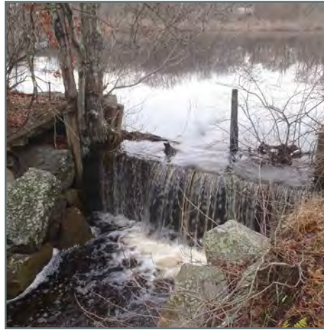
Rattlesnake Brook Restoration Freetown
