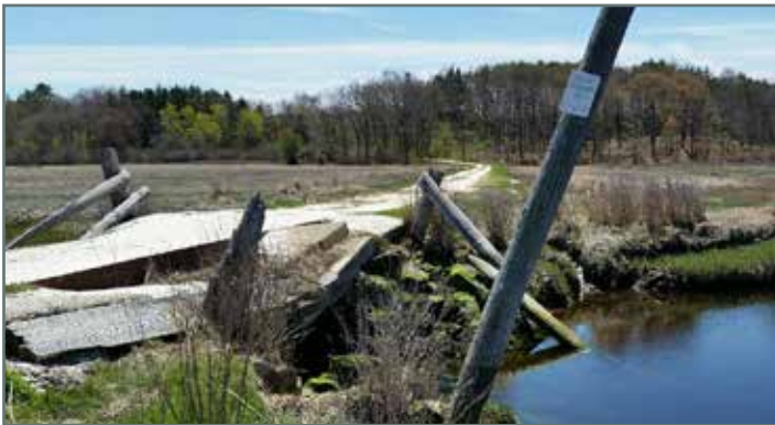
Kent's Island Salt Marsh Restoration, Newbury
