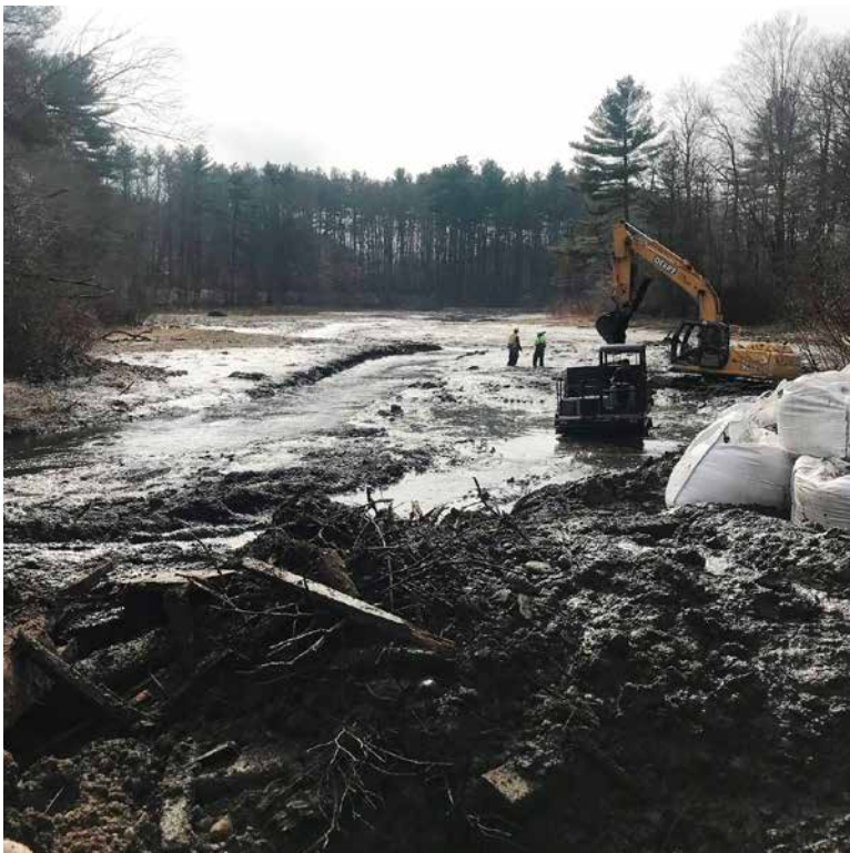
Cotley River, during dam removal and after.
