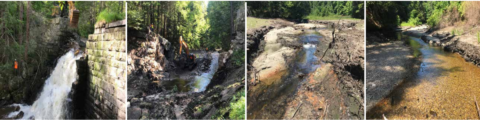
The dam removal and transformation of Upper Roberts Meadow Brook in Northampton.
