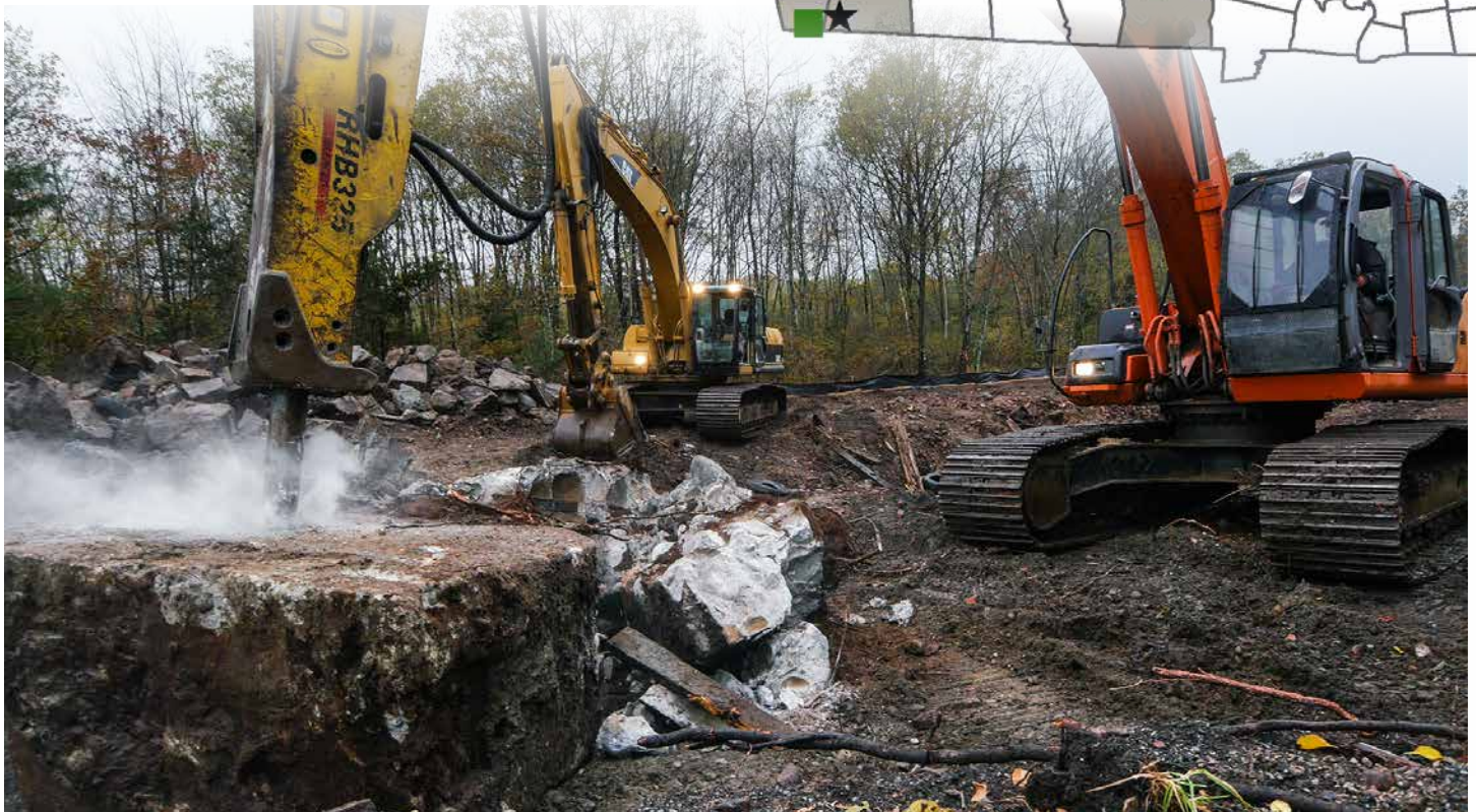
Dam removal in process in Fall River.
