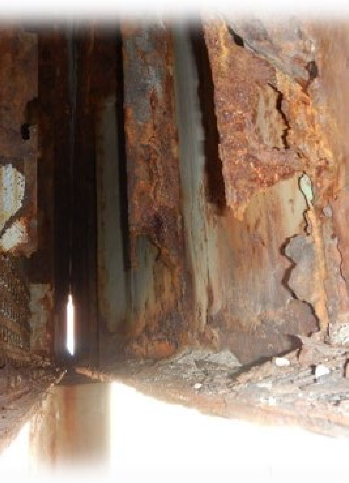
Structural Deterioration – Steel Superstructure
