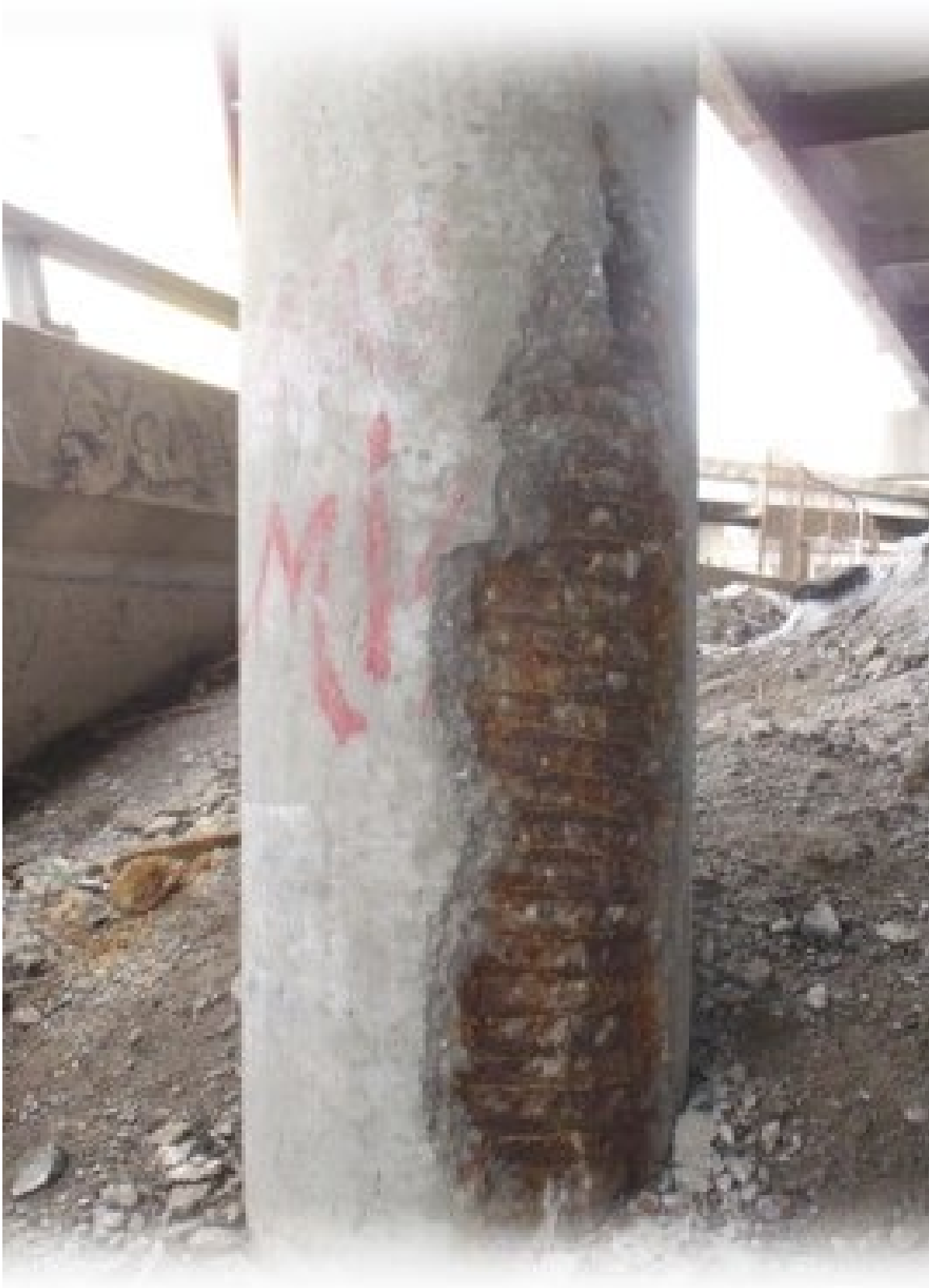
Structural Deterioration – Concrete Substructure
