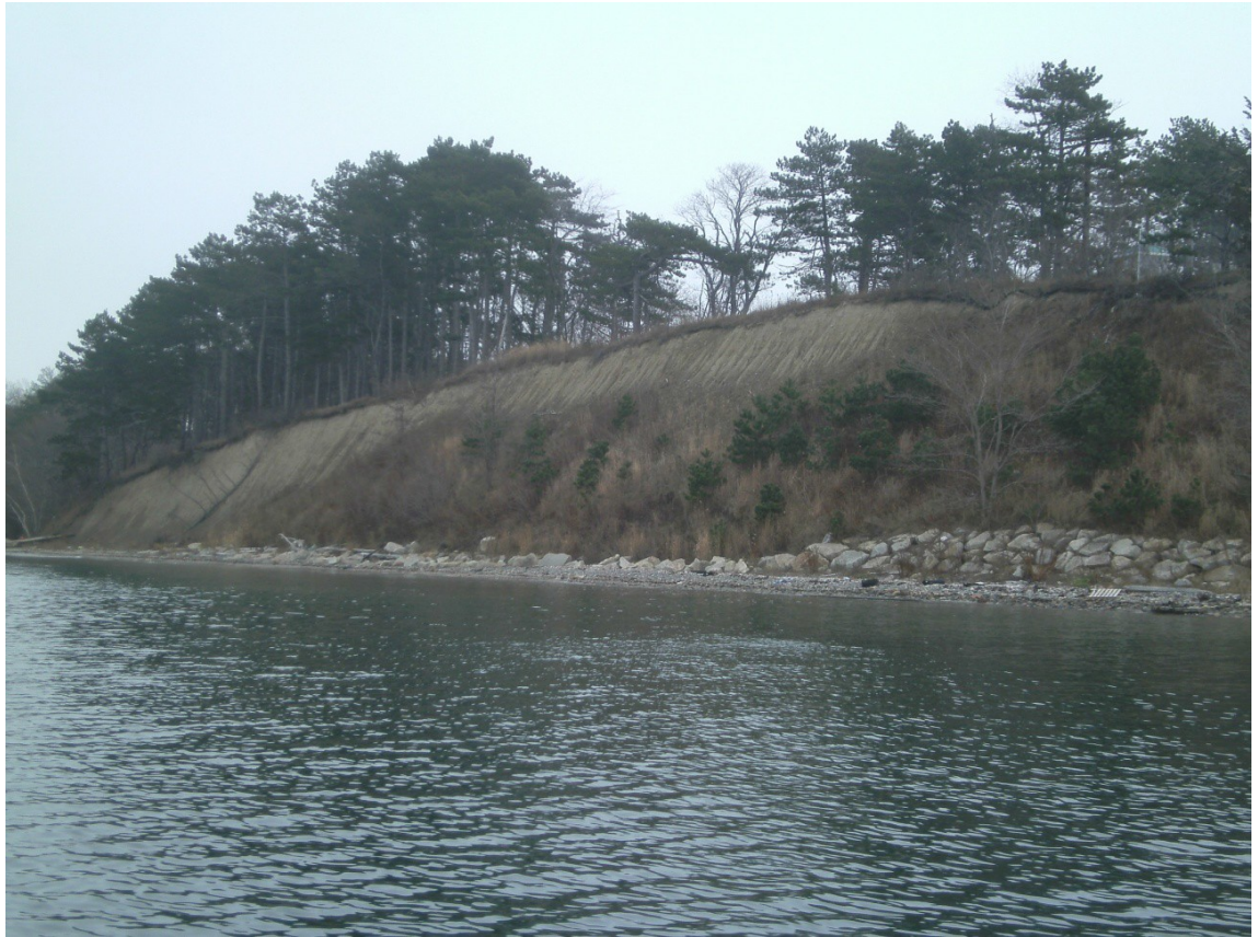
Long Island Shoreline. Sandy/cobble intertidal lined with riprap to support eroding slope
