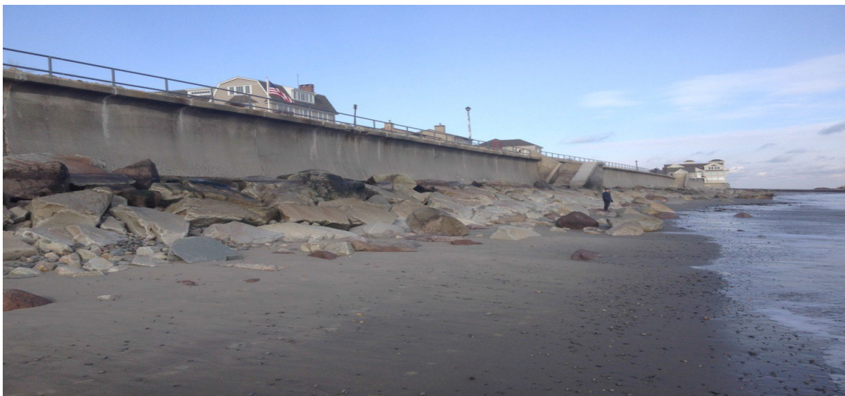
Scituate Bar Rock Shoreline. Note person in front of seawall for reference of size of seawall. Sandy beach in front of riprap and high seawall.
